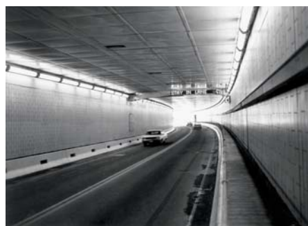
Eisenhower-Johnson Memorial Tunnel in June 1973 shortly after opening
