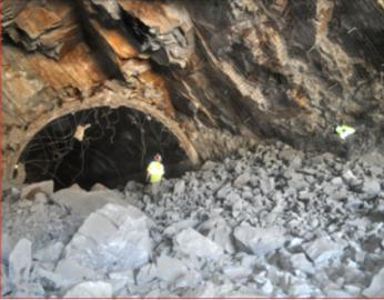
The interior of the eastbound I-70 tunnel bore after a recent blast that advanced excavation 13 feet from the east portal. Crews are 35 percent complete with the tunnel excavation.
