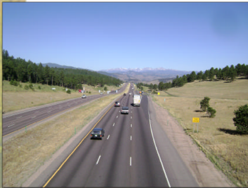
4. View looking west at Genesee
