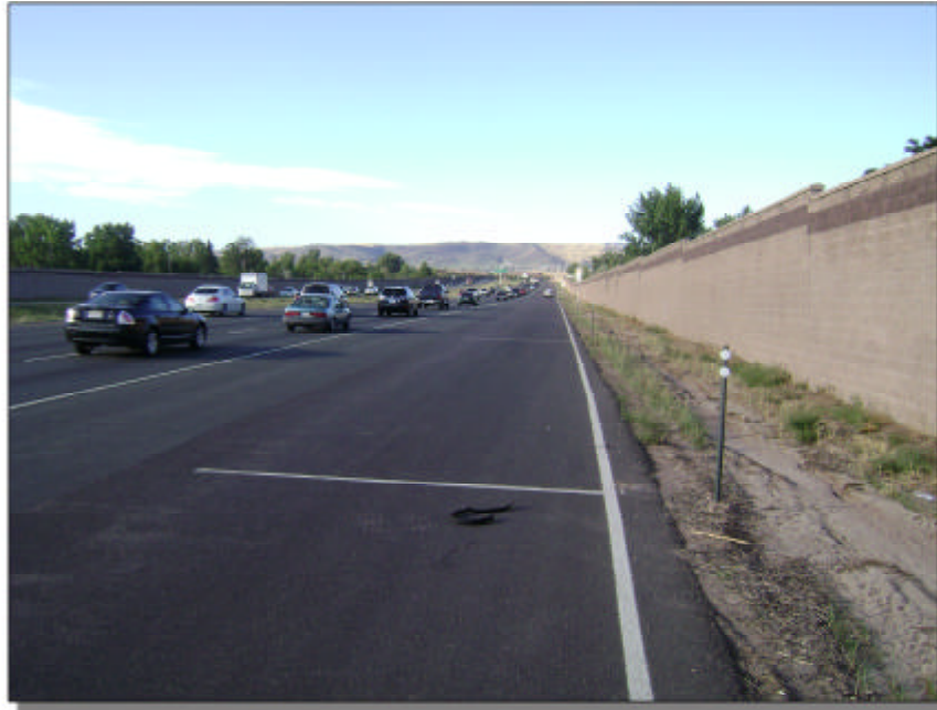
1. View at chain station Exit 263W
