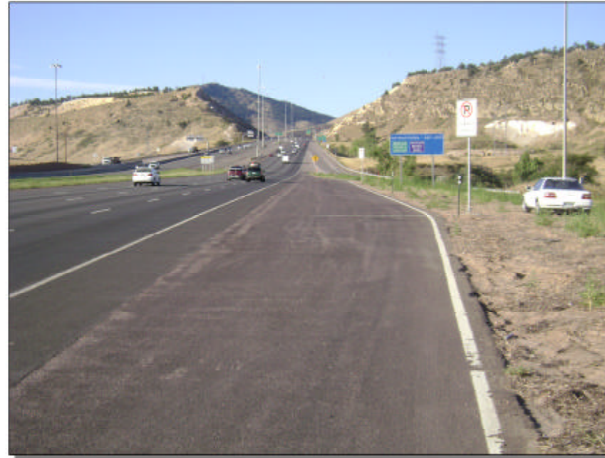
2. View at chain station Exit 260W
