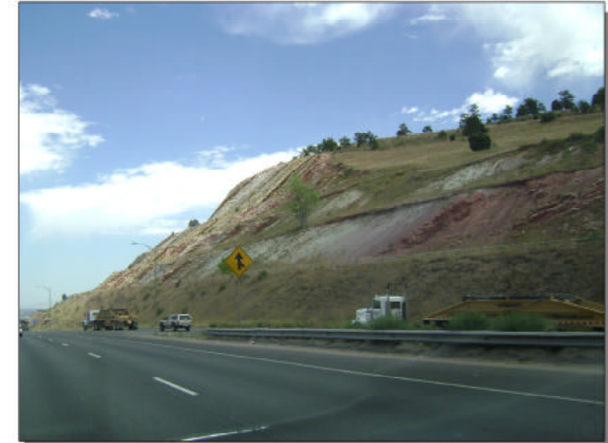
3. Looking north at cut slope
