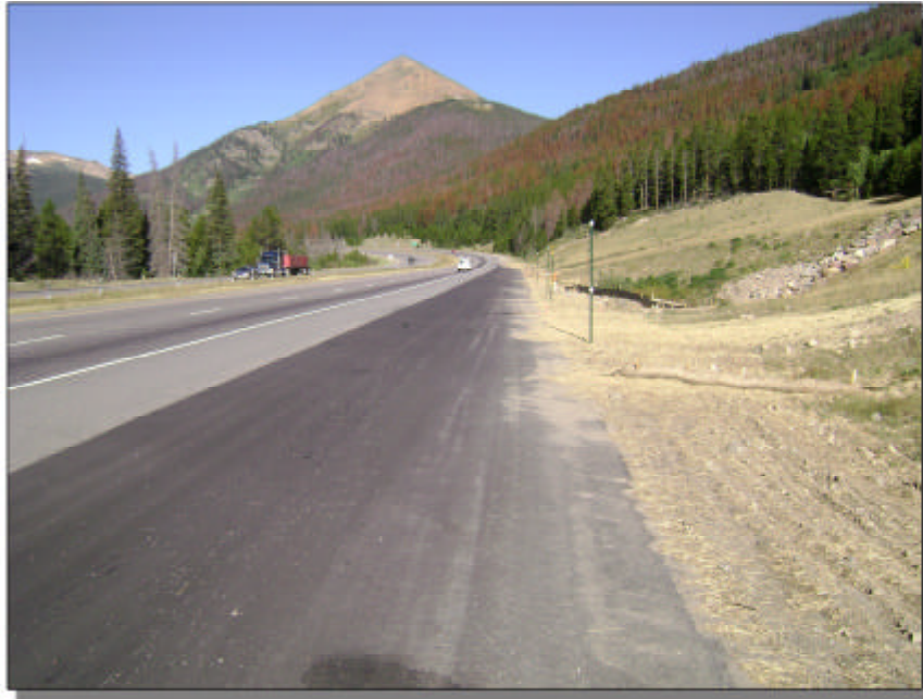
1. View west at chain station Exit 221W
