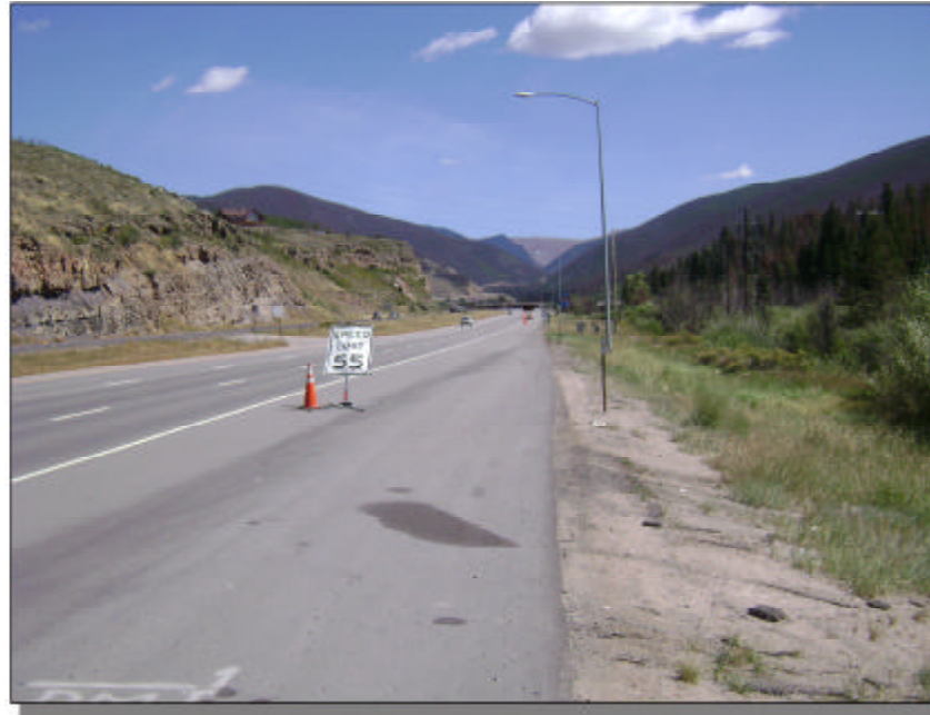
2. View west at chain station Exit 219W
