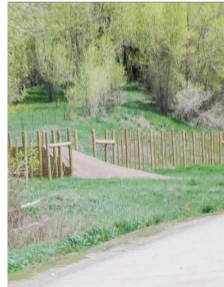
B | Fencing constructed with pressure-treated posts will weather and blend into the landscape.
