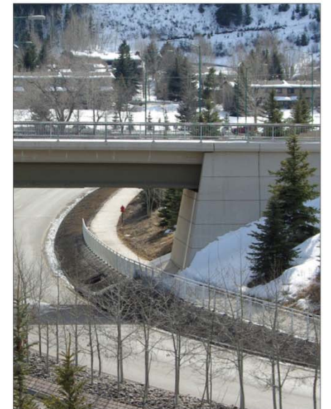
C | Community circulation must be considered at the onset of interchange design to ensure the creation of comfortable pedestrian spaces.
