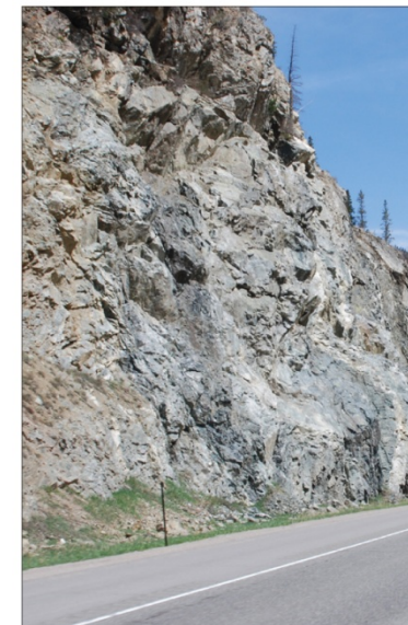
D | Color staining techniques will blend new rock cut with existing rock features.
