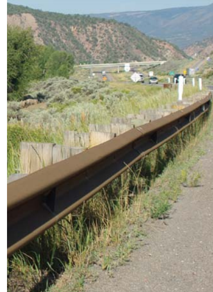
A | Self-weathering Type 3 Guardrail W Beam should be used for guardrails throughout this segment.
