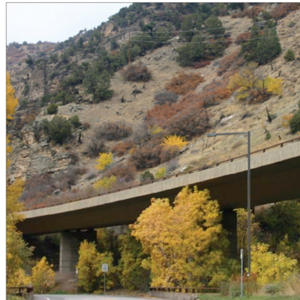
B | The bridge at Grizzly Creek rest area (exit 121) presents an aesthetic character with color, shadow, and box girder construction.
