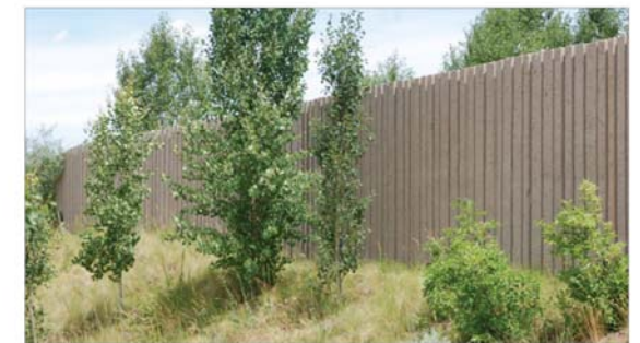
D | When sound walls are required, utilize berming, landscape, texture, and limited wall height.
