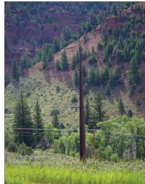
B | Proper color application based on the surrounding natural context blends utility structures into the landscape.
