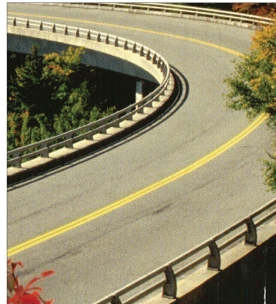
C | Utilizing attached metal rails on bridges rather than concrete barriers adds to the transparency and thin appearance of the span.
