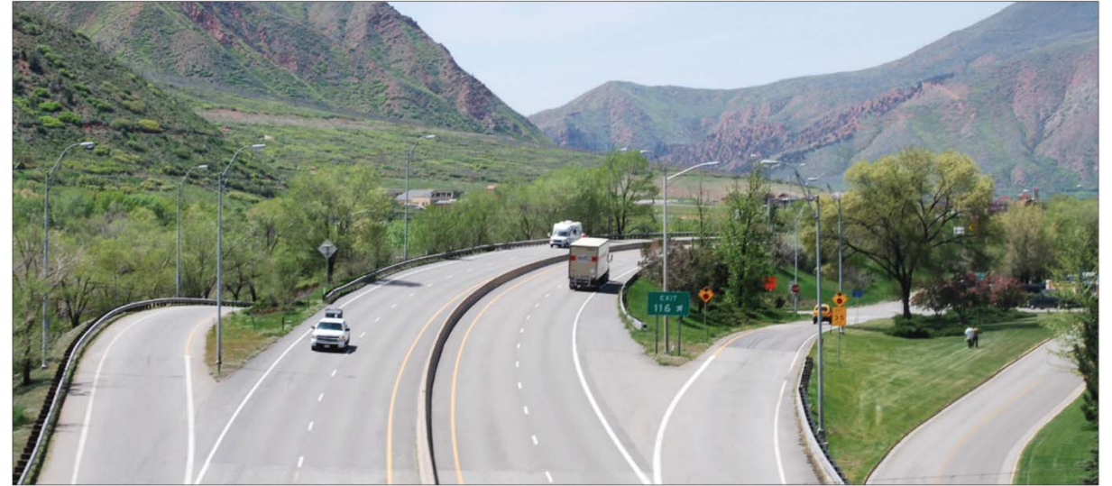
A | Interchanges should exhibit a compact design and include dense landscaping in open areas to create a transition from the transportation corridor to the community environment.
