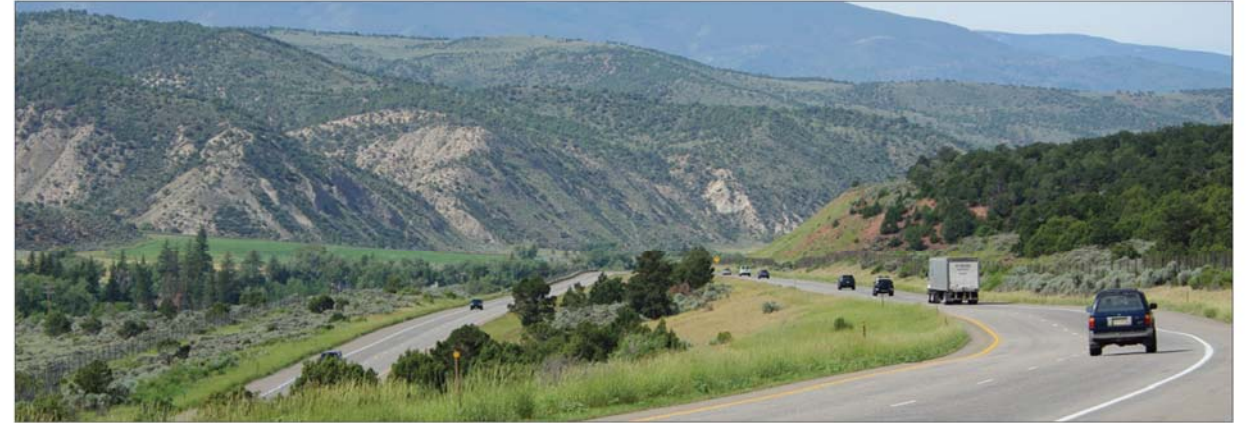
A | Medians of variable width blend the transportation corridor with natural landscape and drainage patterns.
