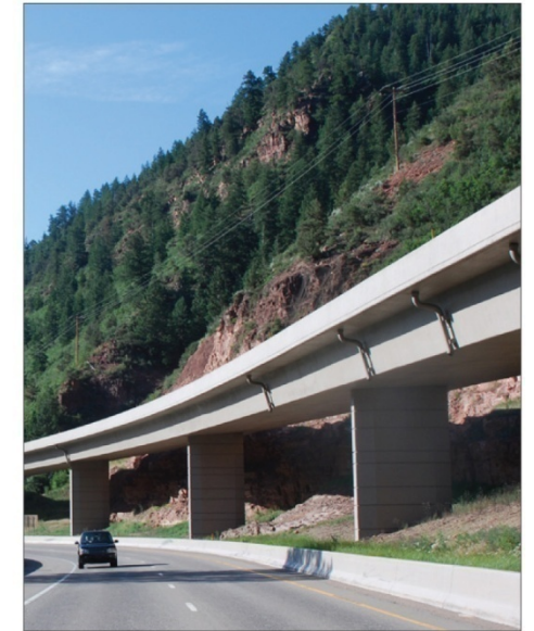
B | Deep overhangs and shadow lines add visual depth and give the bridge superstructure a thin appearance.
