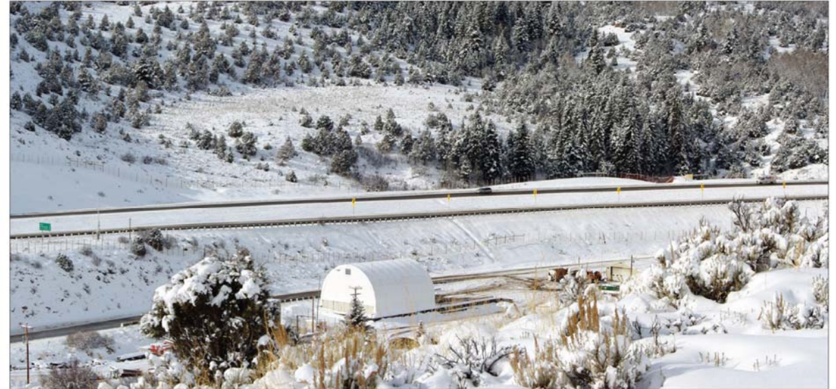
A | The CDOT maintenance facility near Wolcott is often unnoticed by travelers because it is set below the level of the roadway.
