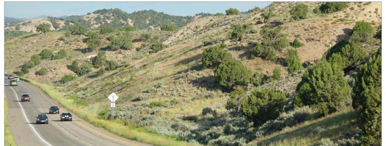
D | Utilizing variable slopes through the length of an embankment mimics the natural patterns found in the alpine landscape.
