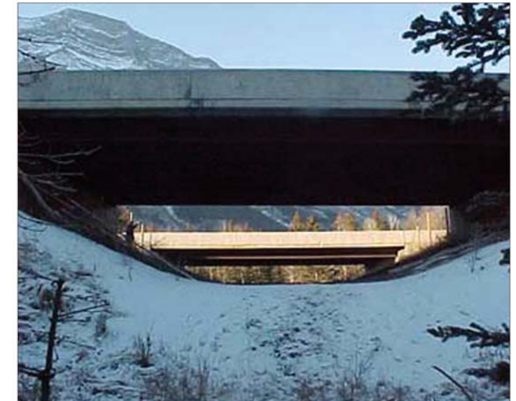
C | Underpasses that utilize open-span bridges offer greater visibility for wildlife than box culverts or enclosed crossings.
