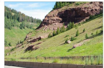
Rock and Earthwork Combined
