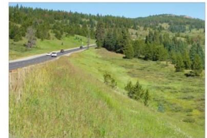
Blended Toe of Embankment
