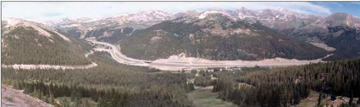
Loveland, view northwest from Loveland Pass along SH 6
