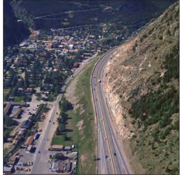
Georgetown, view west
