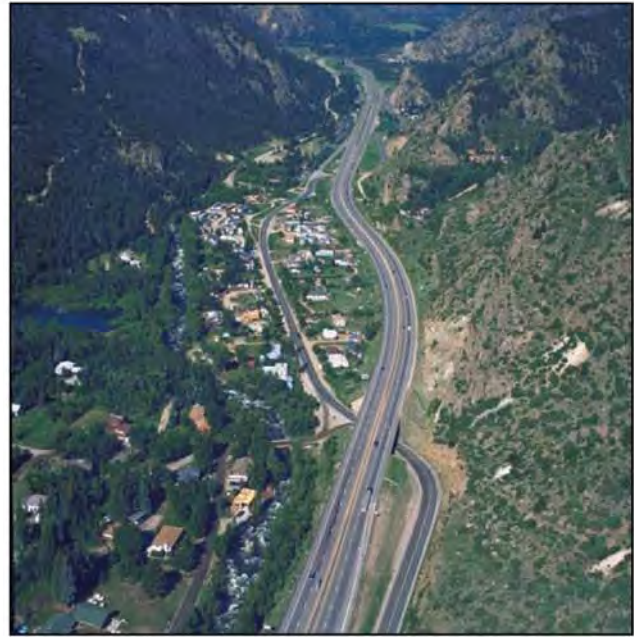
Lawson, view west
