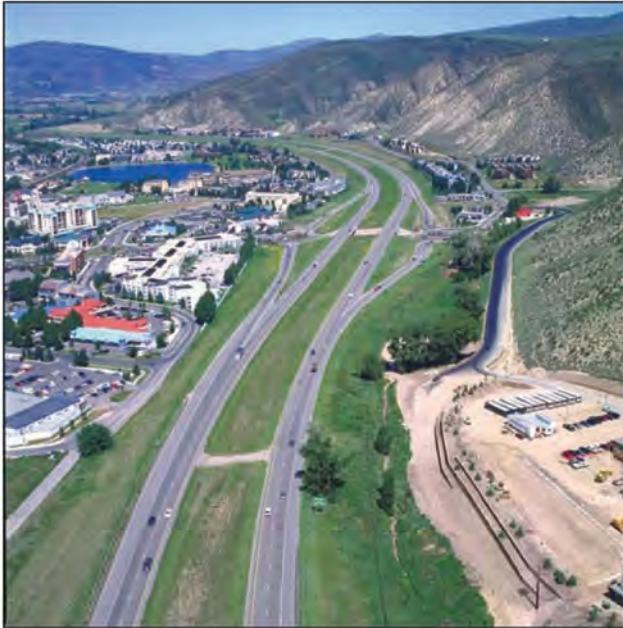
Avon, view west
