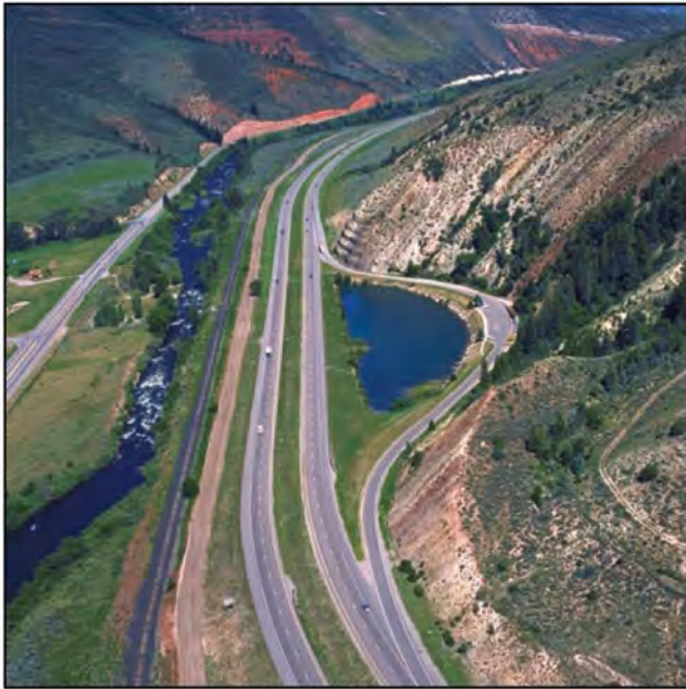
Wilmor Lake, view west
