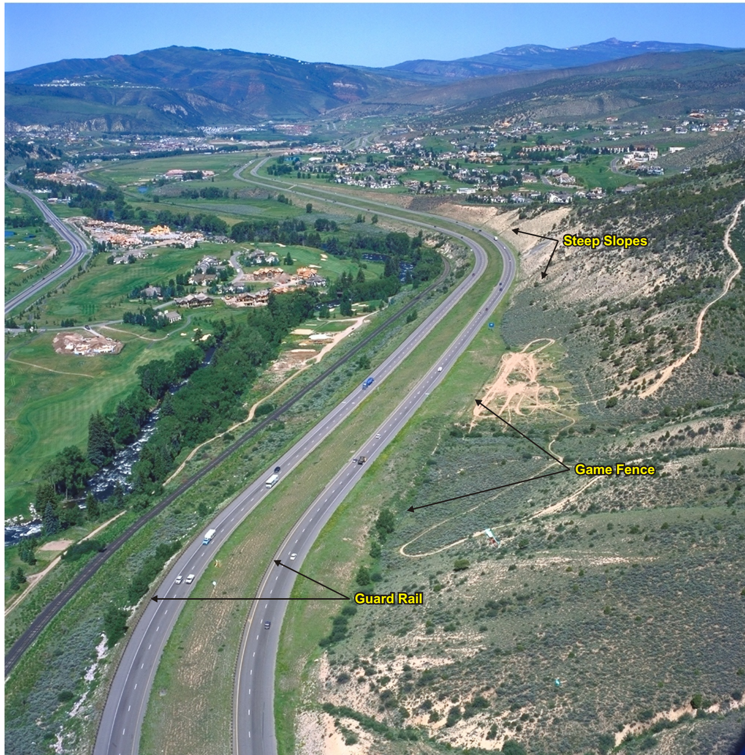
MP 165 westbound, Eagle County
