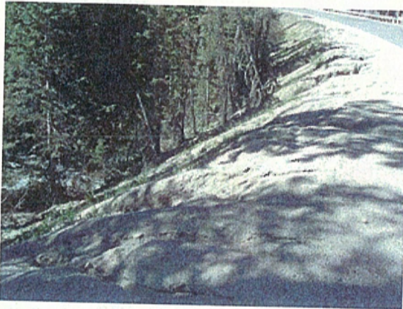
Sedimentation: Clear Creek immediately downstream from Loveland ski area parking; road sand and gravel from US 6.
