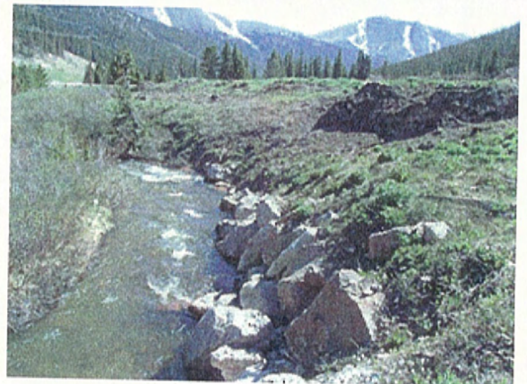
3 Channelization: Channelized Clear Creek immediately downstream from Loveland Valley parking area.
