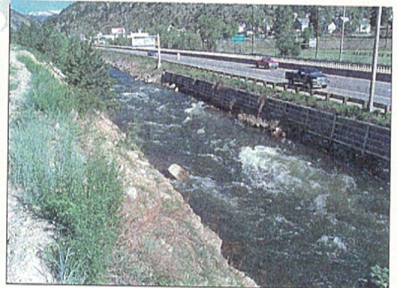
4 Channelization. Clear Creek at Idaho Springs.
