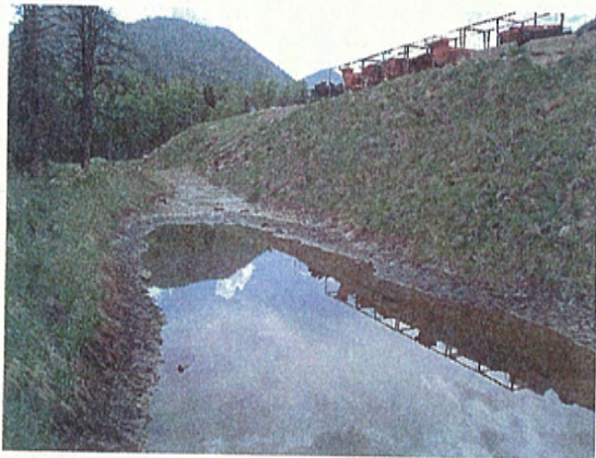
1 Sedimentation/Chemical Deicers. CDOT winter maintenance facility drainage.
