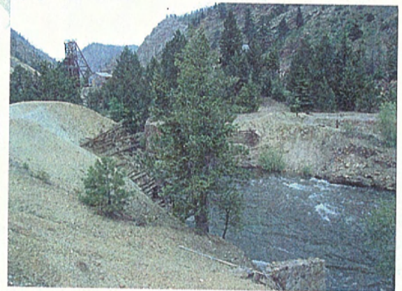
4 Sedimentation/Release of Metals. Donna Juanita Mine materials located on Clear Creek downstream from Dumont.
