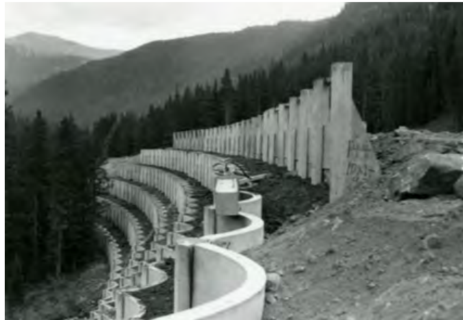
Figure 2. Original Pre-cast Curved Concrete Wall
