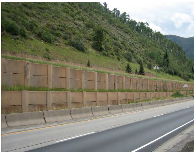
Figure 3. Existing Pre-cast Curved Concrete Wall
