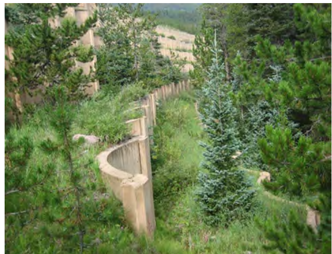
Figure 1. Existing Pre-cast Curved Concrete Wall in Landscape
