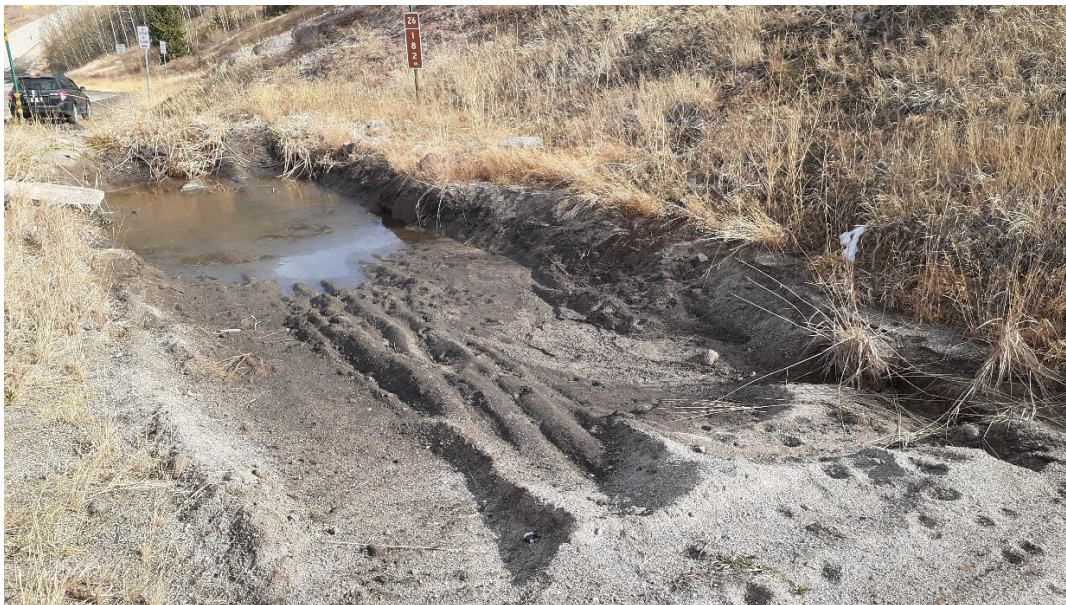
Figure 3.2. Soft-sided Sediment Basin No. 26 on Westbound I-70
