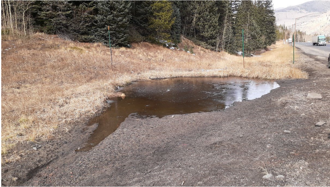
Figure 3.1. Soft-sided Sediment Basin No. 30 on Eastbound I-70
