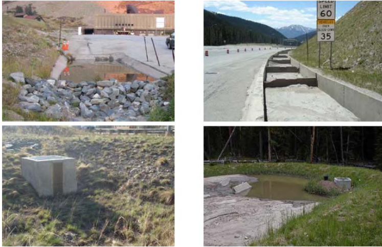
Source: CDOT Clear Creek SCAP, 2013
