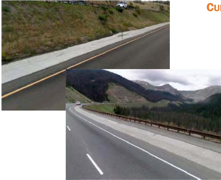
Source: CDOT Clear Creek SCAP, 2013
