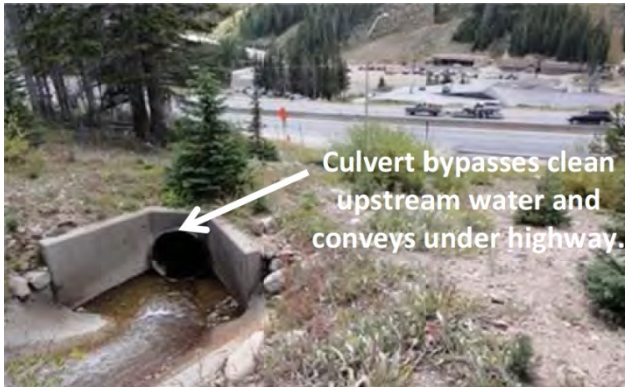
Source: CDOT Clear Creek SCAP, 2013
