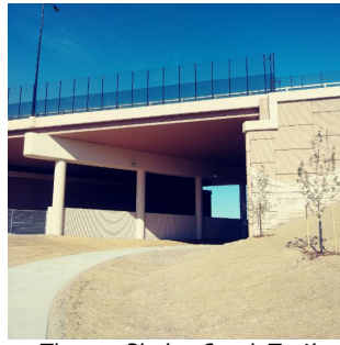
Thomas Phelps Creek Trail under new I-25 bridge
