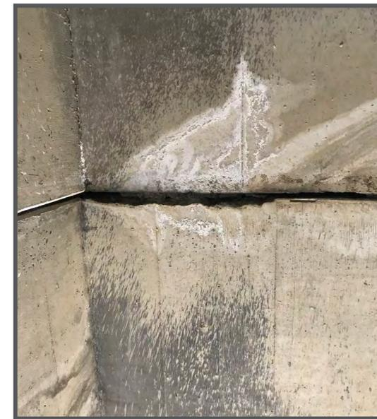
SEPARATION IN CULVERT CEILING
