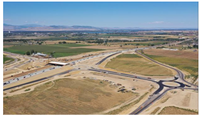
Recent reconstruction of the CO 402 interchange with added roundabouts and Park-n-Ride improvements
