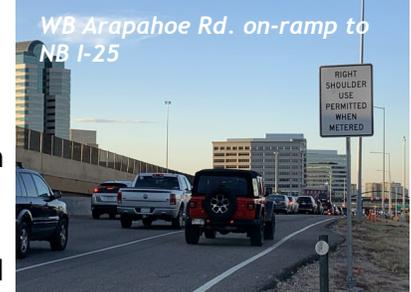
**Early 2022**, the ramp metering system will be extended to I-225 and C-470 on-ramps to northbound I-25. Four ramp metering signals will be at the end of each ramp. Motorists will be able to use the shoulder lanes when the ramp meters are on. New ramp meters will also be activated on the westbound E-470 on-ramp to northbound I-25.
