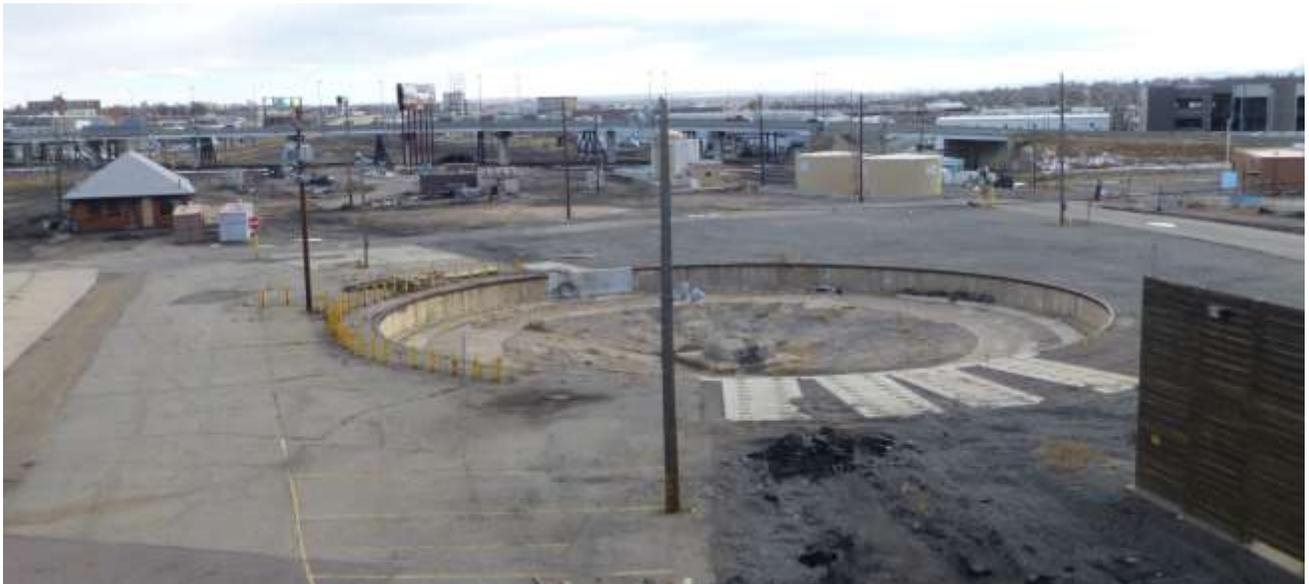
Extant turntable pit marking the location and size of the 1940 turntable, removed in 2016. Photo by James Steely, 2016.
