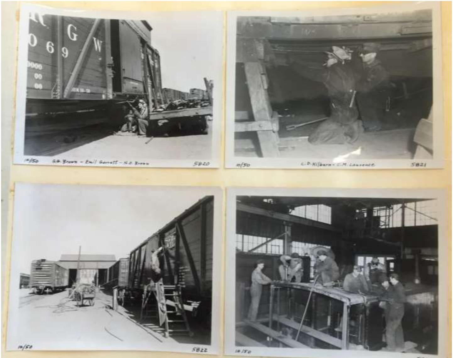
Burnham Shops 1950, Photos Showing a Variety of Shop Work, Clockwise from Upper Left: Repairs to Box Car Underframe; Brake Repairs to Box Car; Stenciling of Logo to Box Car (Wood Car Shop in Background, Not Extant); Constructing a Caboose Cupola inside the Steel Car Shop (Extant)
