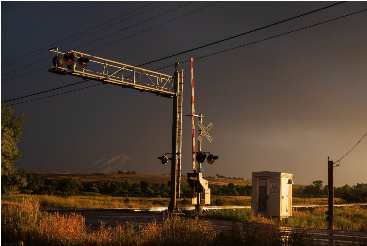
Figure 23: Grade Crossing in Craig, CO
