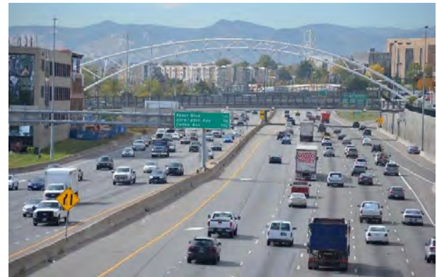
I-25 looking south from the 20th Street bridge
