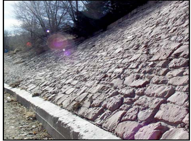
WPA Flood Wall Along Monument Creek
