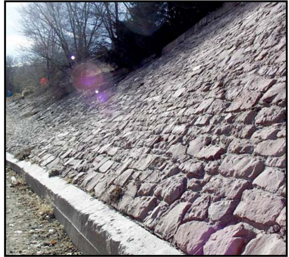
WPA Flood Wall Along Monument Creek
