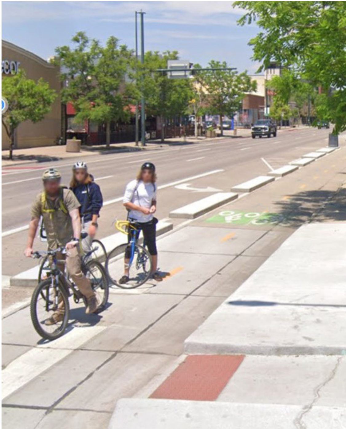
Concrete curb-protected two-way bike lane.
