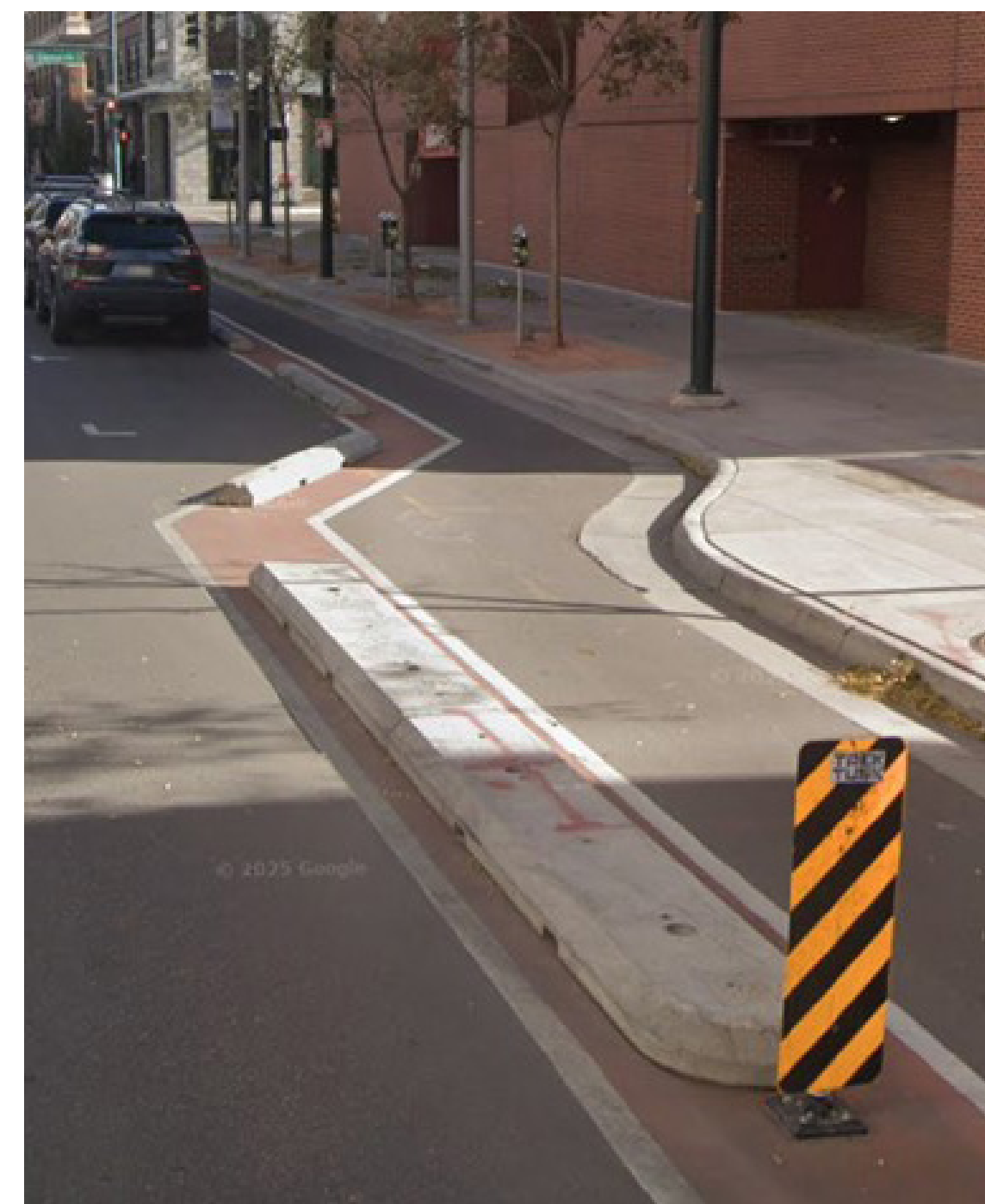
Concrete curb-protected bike lane with colored buffer.
