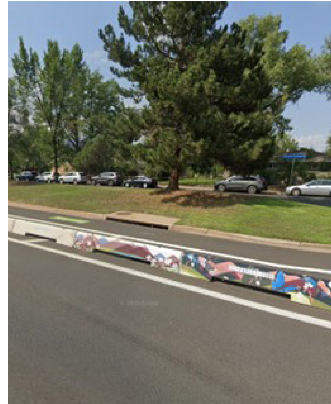
Concrete barrier with striped buffer-protected bike lane. Painted barrier makes the design more aesthetically pleasing.
