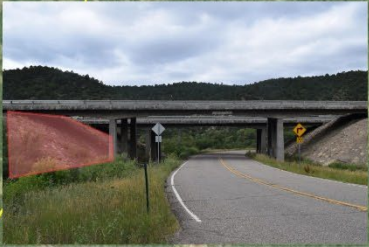
Removing the slope under the bridge and adding a wall were considered, but because of the high cost of construction and unlikelihood of animal use, this idea was not advanced.
