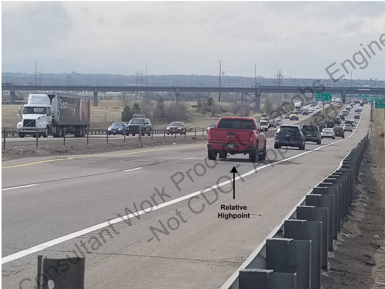
1 2 Figure 2-13. Differential Settling Between South Platte River and Brighton Boulevard 3 Source: Jacobs
