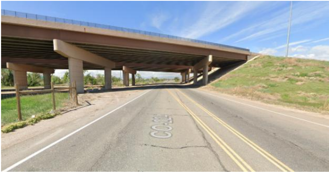
Figure 11. CO 224 Crossing Under I-270, Looking East
