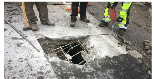
Bridge deck failure on I-270 over the Burlington Ditch
