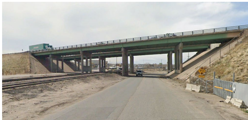
Figure 2-14. East 60th Avenue and BNSF Under I-270 Looking South
