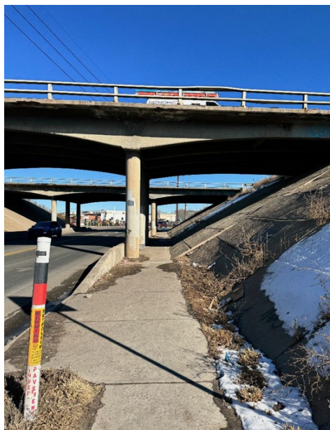
Figure 2-16. East 56th Avenue at I-270 Looking Northbound
