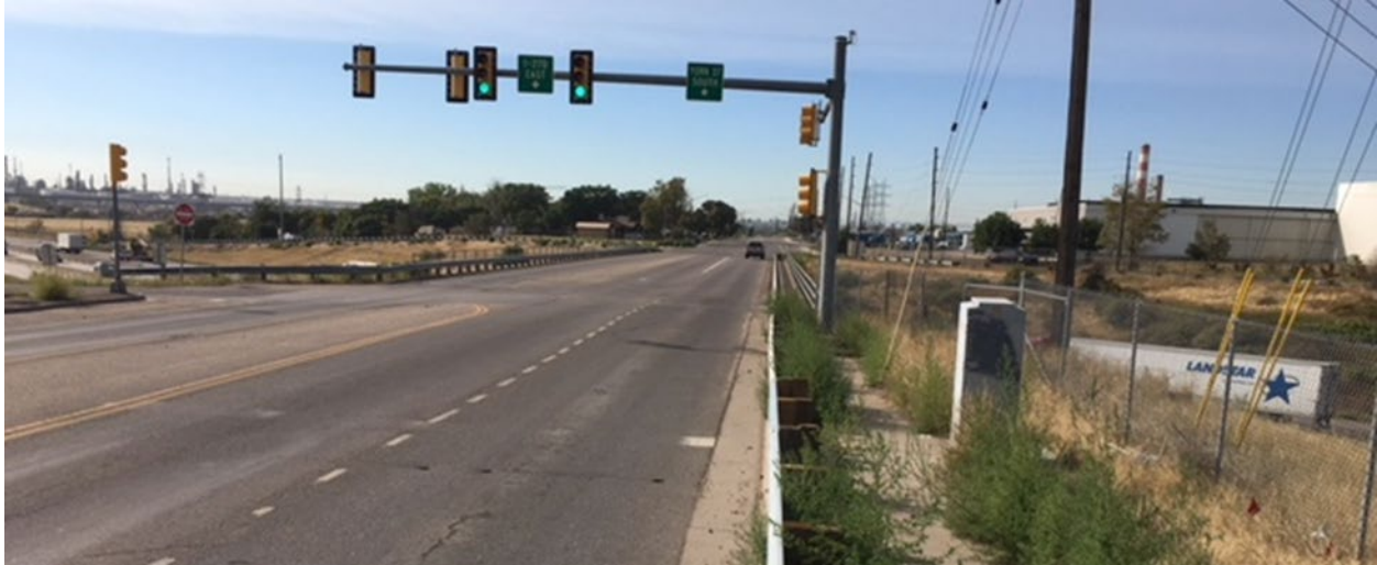
Figure 2-10. York Street at I-270, Looking Southbound
