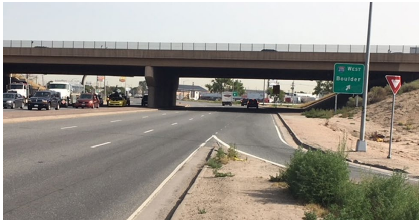
Figure 2-15. Vasquez Boulevard at I-270 Looking Northbound
