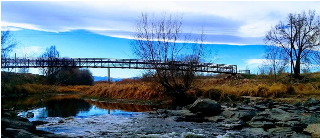
Figure 2-11. South Platte River Trail Bridge Over Clear Creek (Source: Google Maps)
