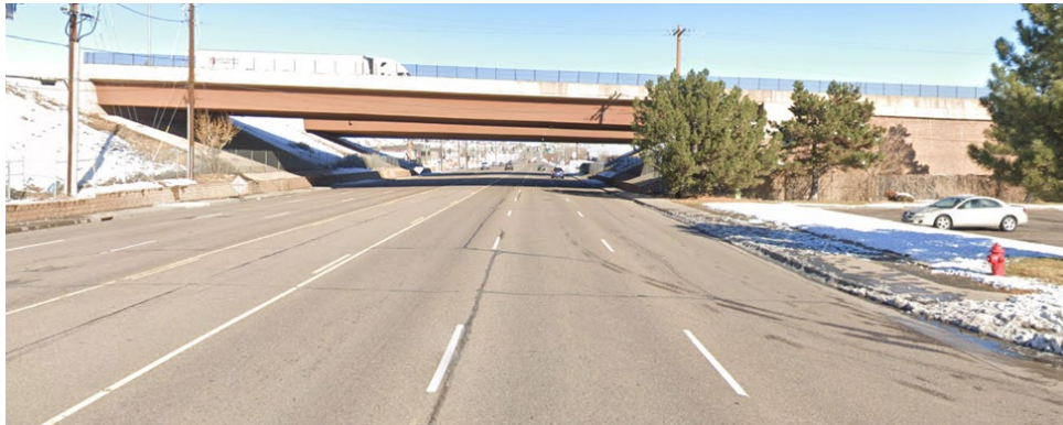
Figure 2-8. Washington Street at I-270 Looking Northbound
