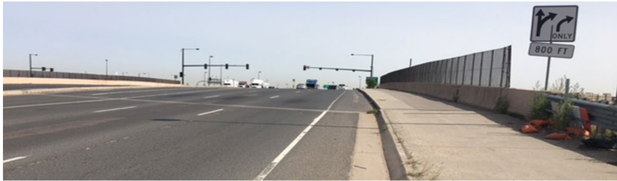
Figure 2-17. Quebec Street Over I-270 Looking Northbound
