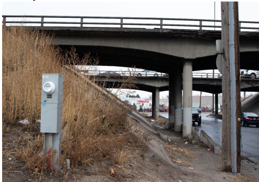
Figura RE-6. Cruce Cajo I-270 en 56th Avenue
