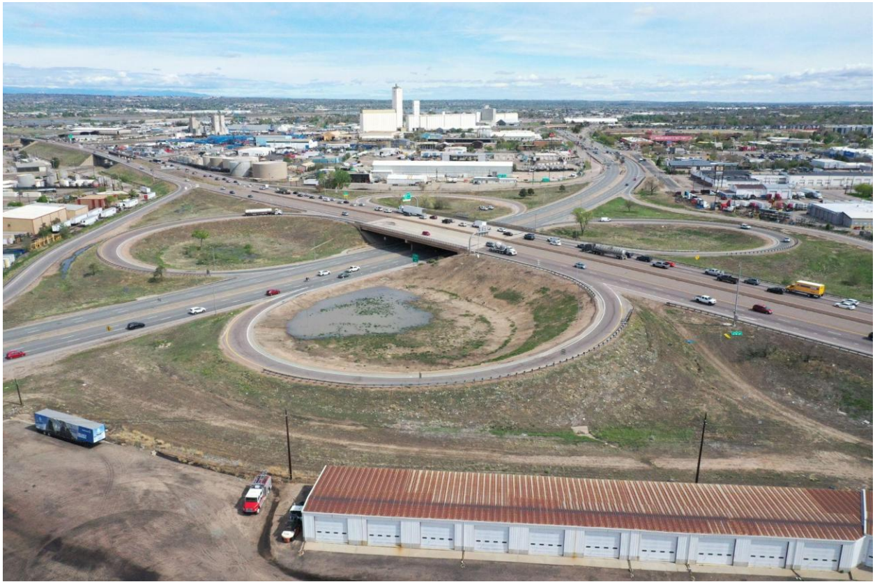
I-270 and Vasquez Boulevard interchange with industrial and commercial development surrounding the interchange, facing north.
