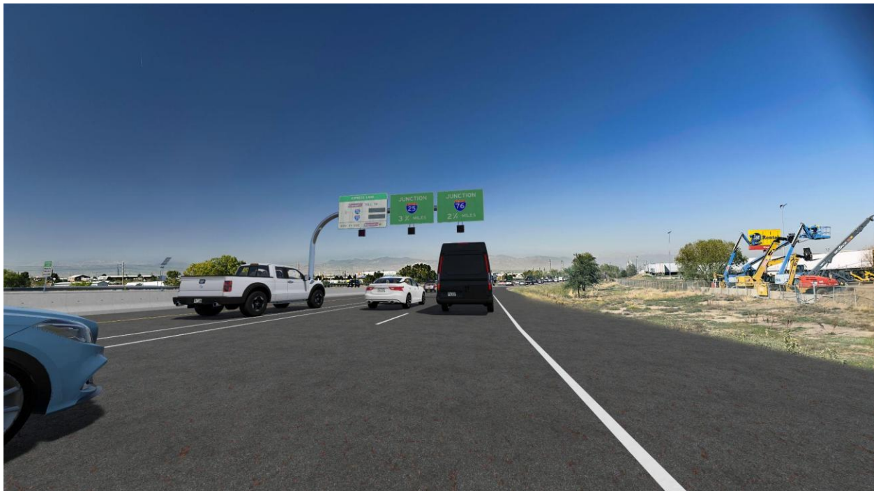
Figure 12. Two General-Purpose Lanes and One Express Lane that Accommodates Transit Alternative Configuration
