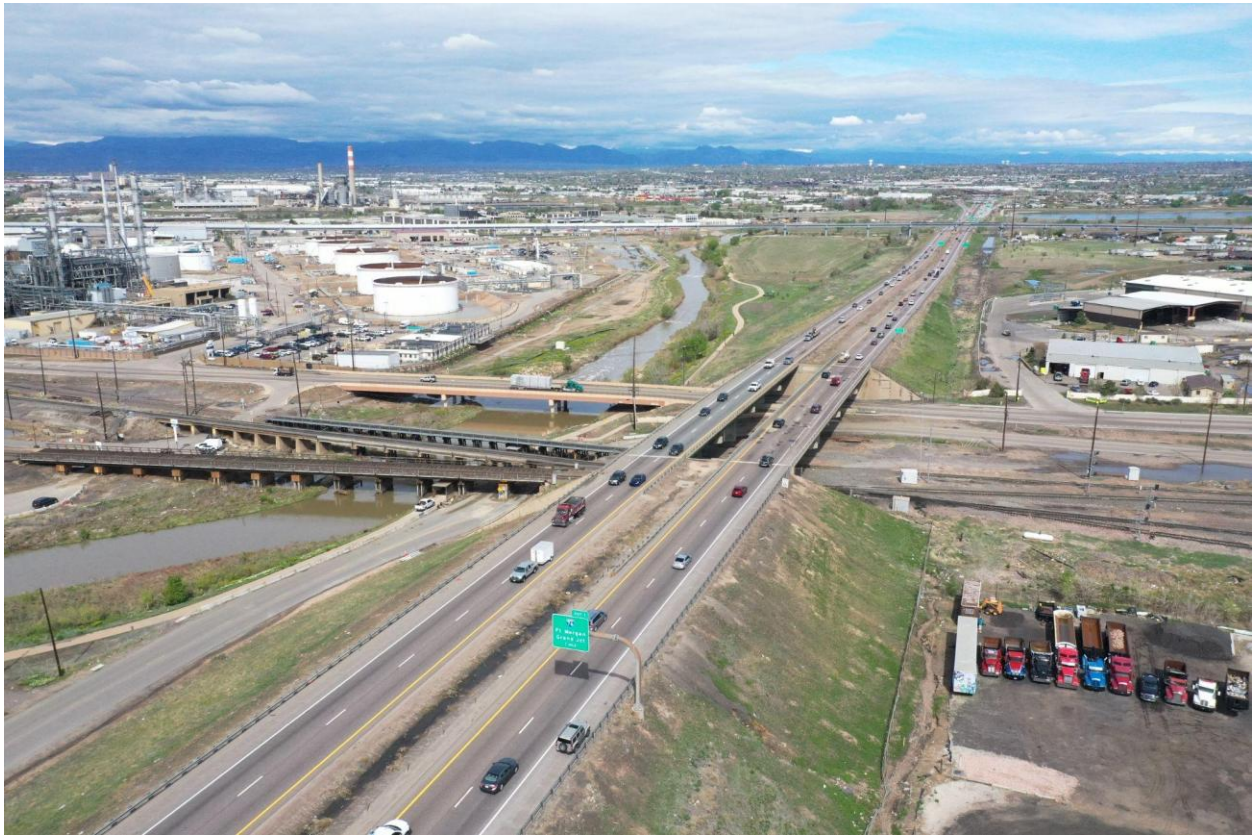
I-270 crossing over the BNSF and UPRR railroads and Brighton Boulevard. Sand Creek and the Sand Creek Greenway trail run along the south side of I-270. Industrial development surrounds the highway, facing northwest.
