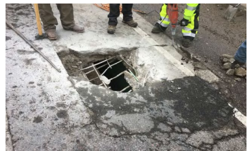
Bridge deck failure on I-270 over the Burlington Canal
