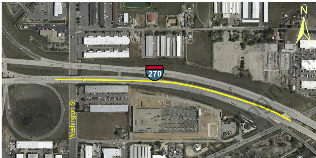
Figure 22. Summary Section - Eastbound from I-25 to I-76 (270B 0.17-0.67)
