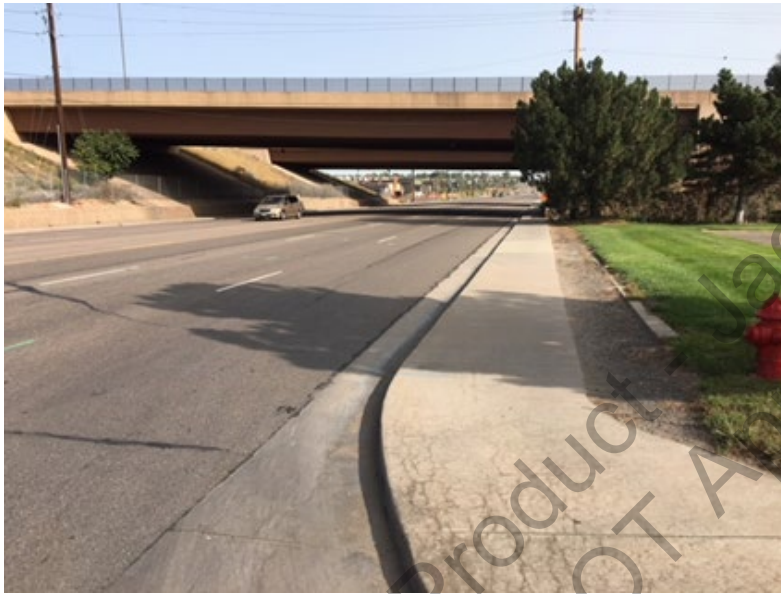
Figure 4-7. Washington Street Washington Street under I-270 looking north. Source: ACL Engineering
