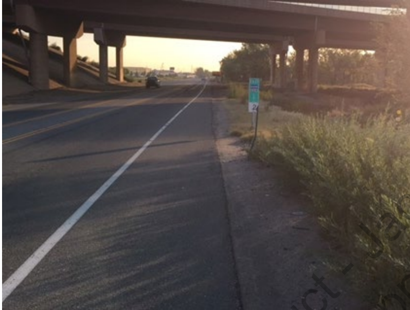
Figure 4-9. 70 th Avenue (SH 224) 70 th Avenue (SH 224) under I-270 looking east. Source: ACL Engineering
