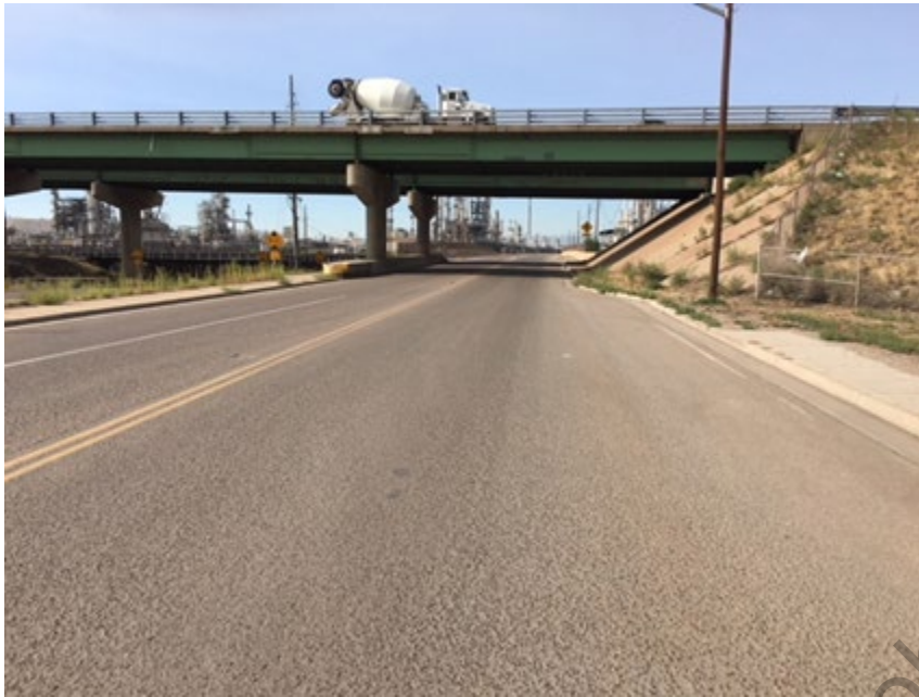
Figure 4-13. Brighton Boulevard Brighton Boulevard crossing I-270 looking south. Source: ACL Engineering
