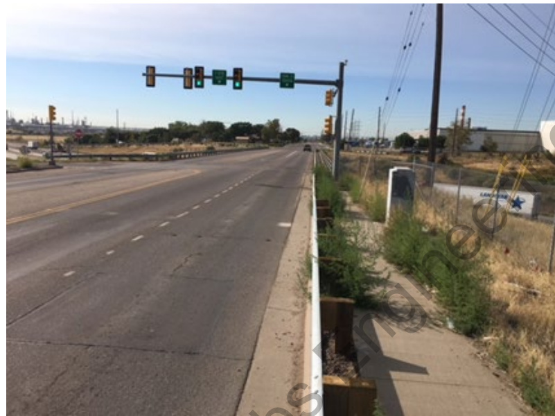
Figure 4-11. York Street York Street Crossing I-270 Looking South Source: ACL Engineering
