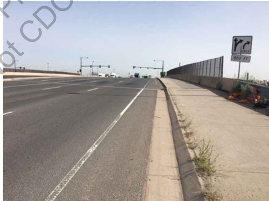
Figure 4-20. Quebec Street Quebec Street crossing I-270 looking north. Source: ACL Engineering
