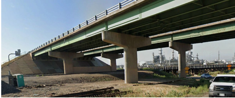
Figure 4-5. Piers and Pier Protection Wall within the Railroad Right-of-Way
