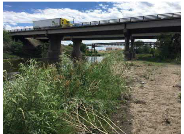
W231 — View of W231, looking southwest.
