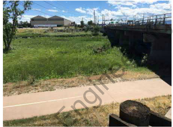
W050 — View of W050, looking southwest.
