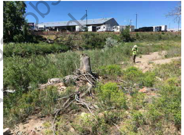
W027 — View of W027, looking west.
