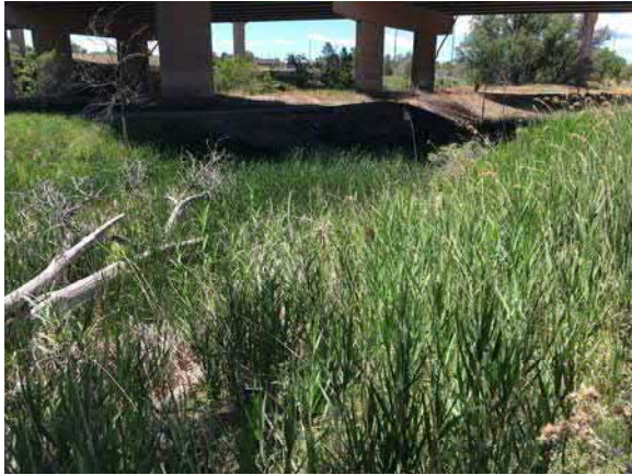
W200 – View of W200, looking south.
