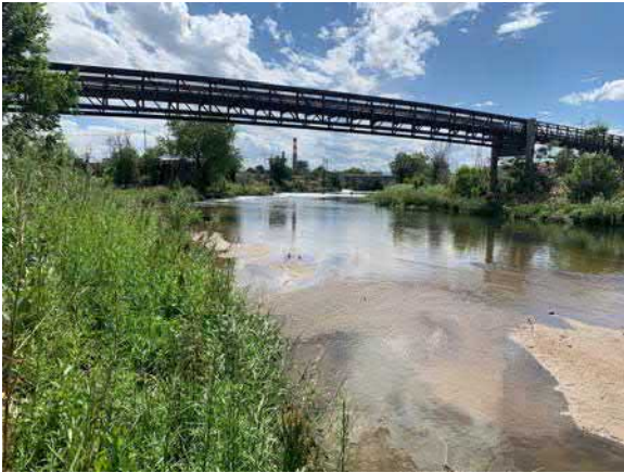
W232 — View of W232, looking southwest.
