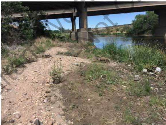
W230 — View of W230, looking northeast.
