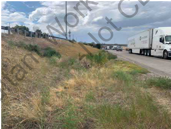
W440 — View of W440, looking northwest.
