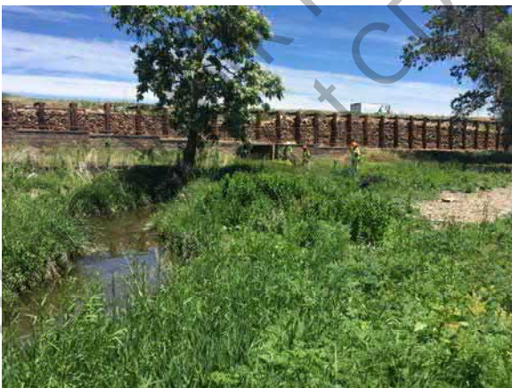
W030 — View of W030, looking northeast.
