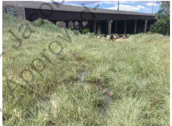
W003 — View of W003, looking southwest.
