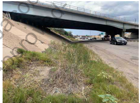
W430 — View of W430, looking northwest.
