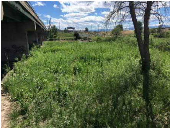
W051 - View of W051, looking southwest.
