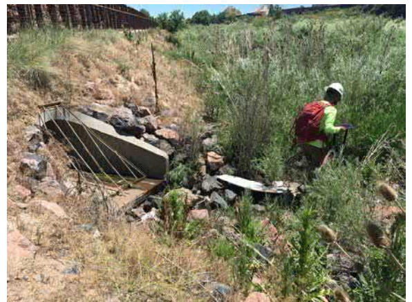
W031 — View of W031, looking southeast.
