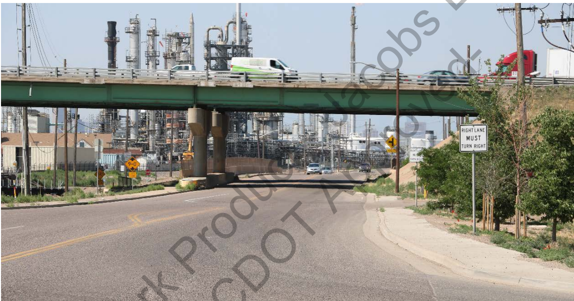
Figure 82. View of Brighton Boulevard/SH 265 at Colorado Boulevard looking at I-270, view facing southwest. The existing I-270 three-span bridge structures would be replaced with a wider, two-span, single structure that spans the highway right-of-way. No improvements would be made to the roadway within the historic boundary.
