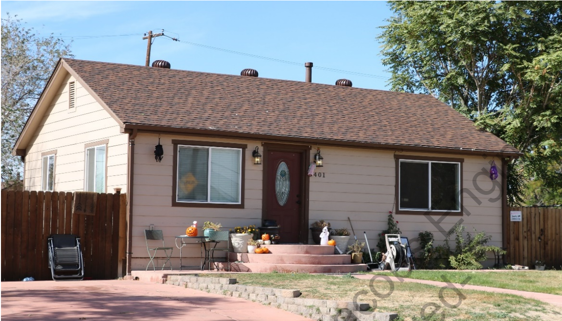
Figure 60. The Colombo House, front (east) elevation. View facing northwest.
