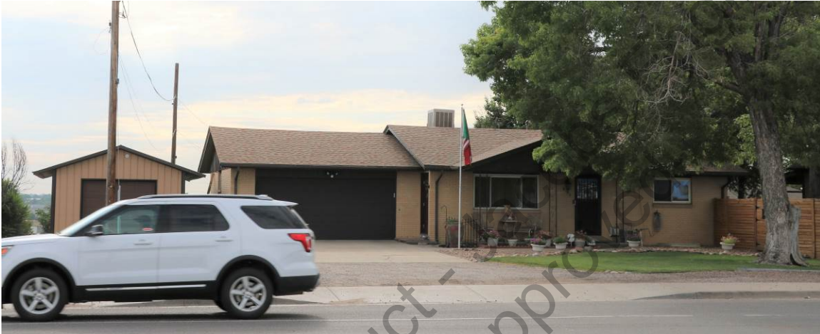
Figure 32. Chapman-Depinto House, front (west) facade and side (north) elevation. View facing east/southeast.
