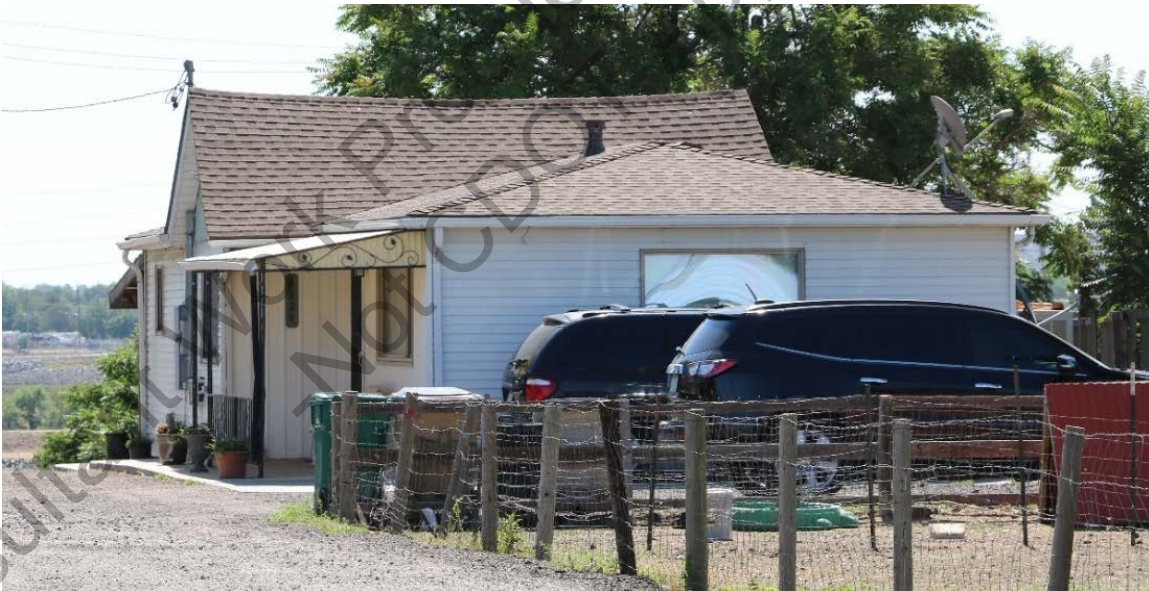
Figure 47. 6824 Columbine Street facade (north) and west elevation, view facing southeast. The original house had vertical painted wood siding, visible under the front awning.
