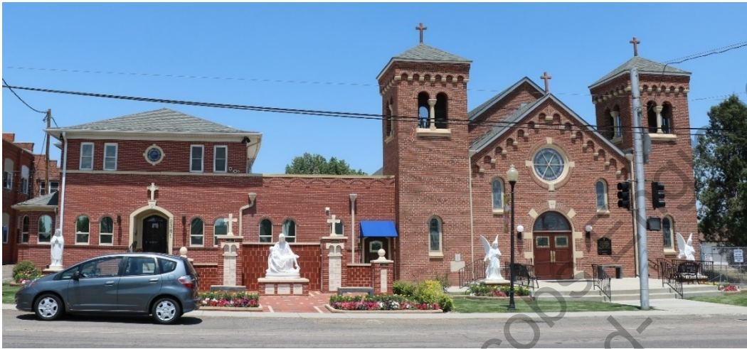
Figure 6. Assumption Roman Catholic Church and rectory currently located at 2361 E. 78 th Avenue in Welby. Mead & Hunt, Inc., 2020.
