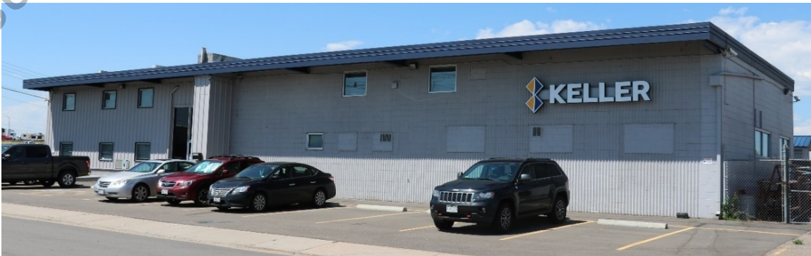
Figure 57. 5775 Eudora Street (Building A), view facing southwest (facade).
