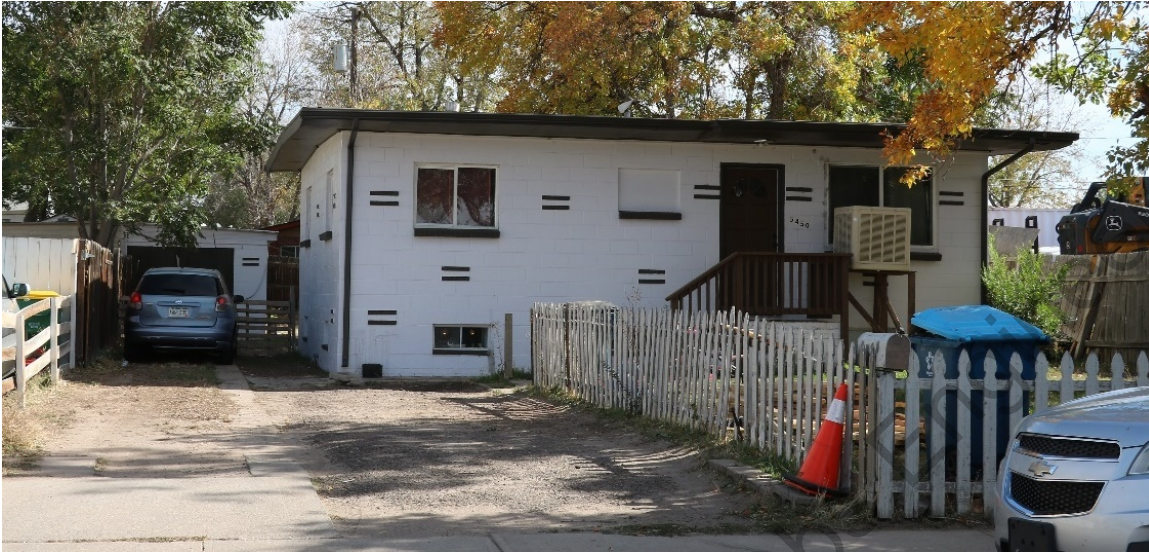
Figure 58. The house at 5450 Krameria Street, front (west) elevation. View facing east.
