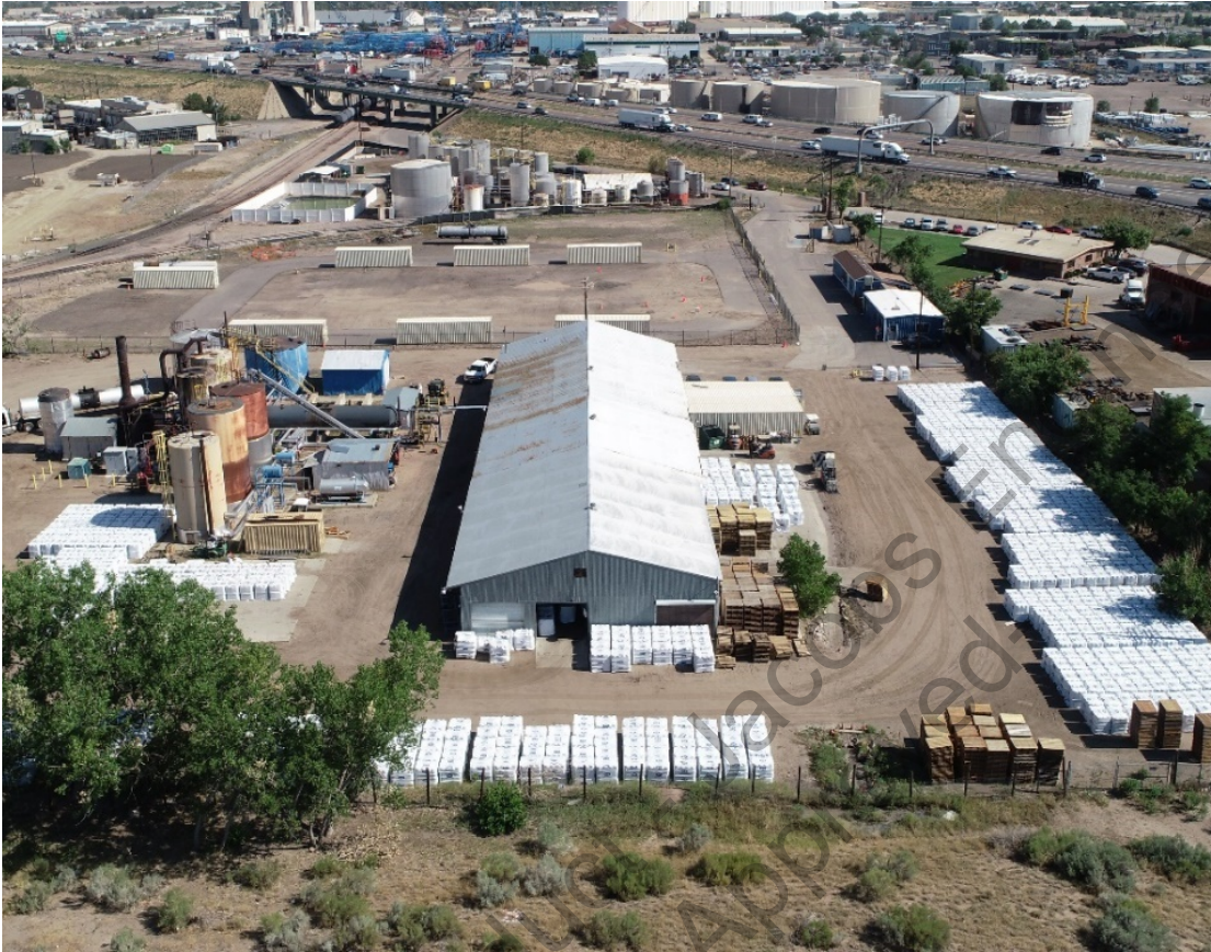
Figure 49. 4303 E. 60 th Avenue, view facing north. Photo from the Colorado Department of Transportation.
