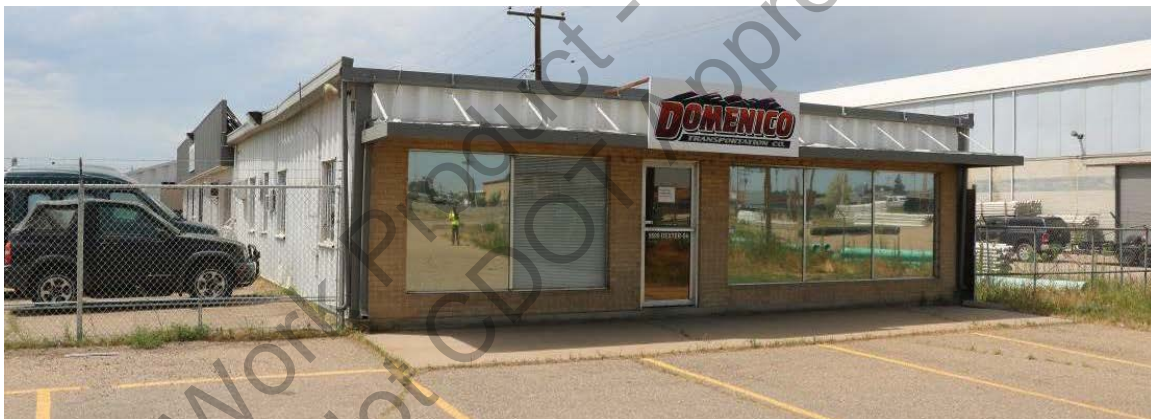
Figure 39. Domenico Transportation Services Building, front (east) facade and side (south) elevation. View facing northwest.
