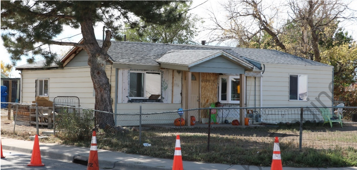
Figure 62. The Duran House, front (north) elevation. View facing southwest.
