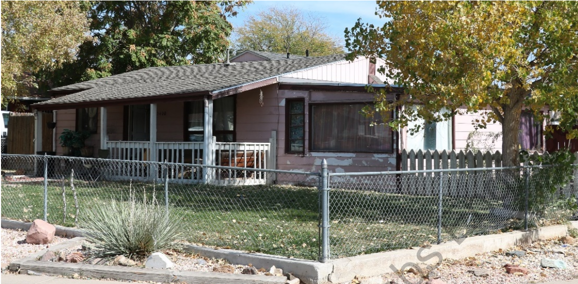
Figure 59. The Hernandez House, front (west) elevation. View facing northeast.
