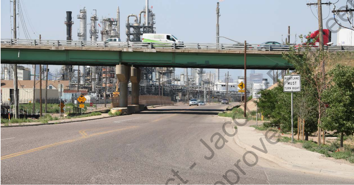
Figure 70. Brighton Boulevard/SH 265 at Colorado Boulevard looking at the terminus of the segment beyond the I-270 overpass. View facing southwest.
