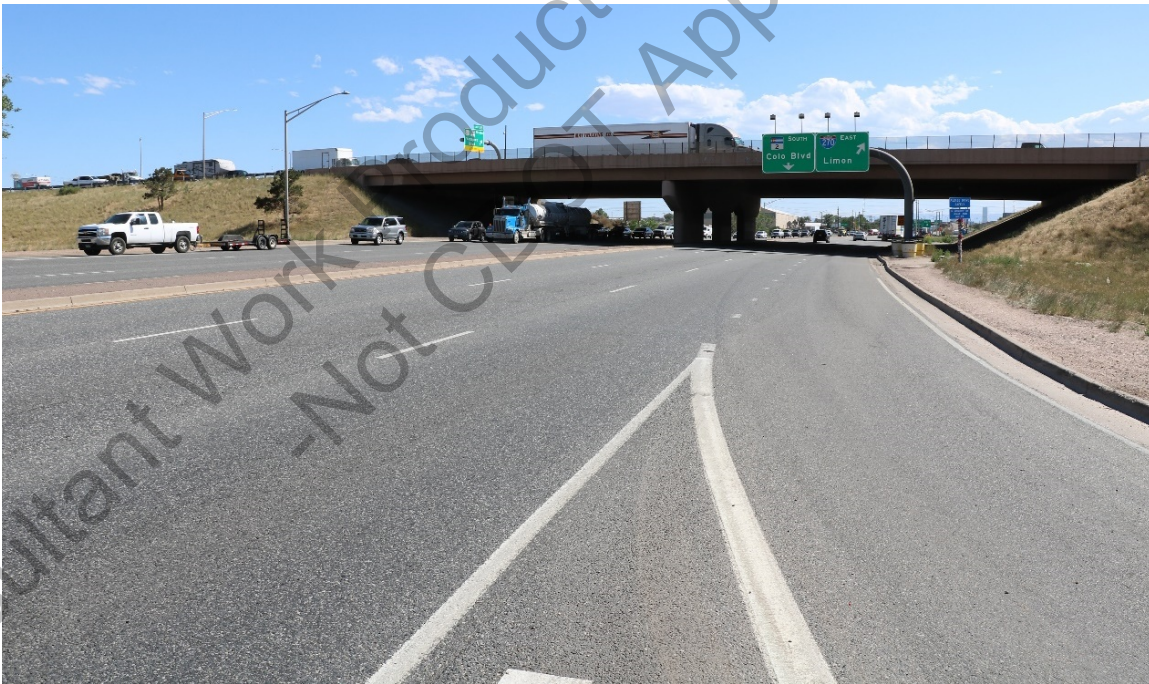
Figure 71. The north terminus of Segment 5AM.3924.2 at Vasquez Boulevard/US 6/US 85/SH 2 and I-270, view facing southwest.
