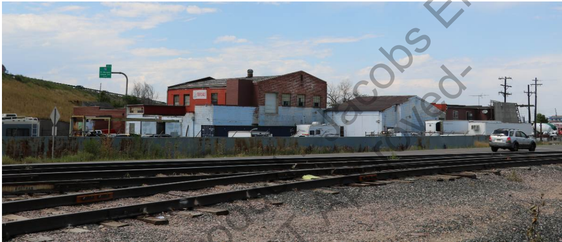
Figure 38. Main building at Denver Oil, side (east) and rear (south) elevations. View facing west/northwest.
