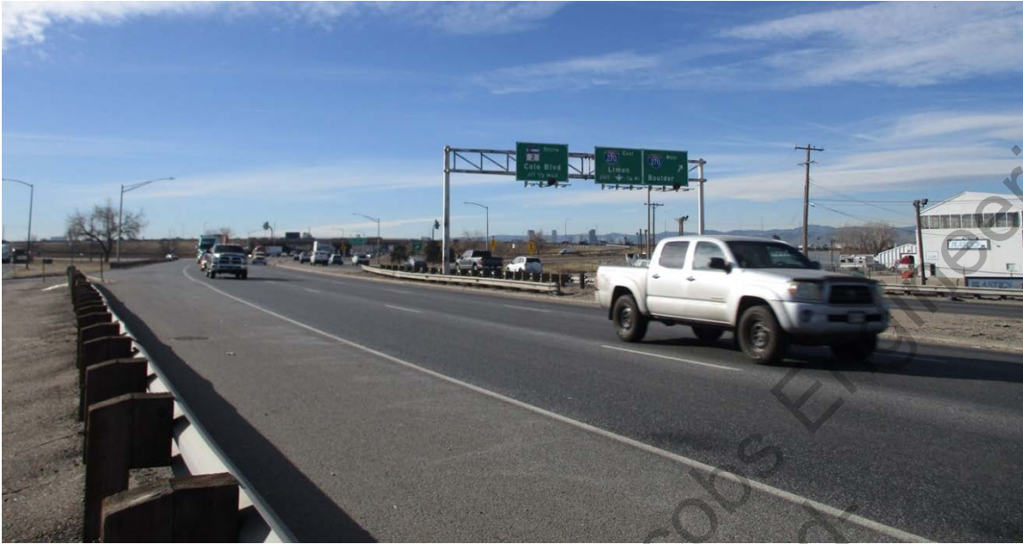
Figure 72. Looking southwest at US 6 (5AM.3924.3) near project's southern terminus at I-270
