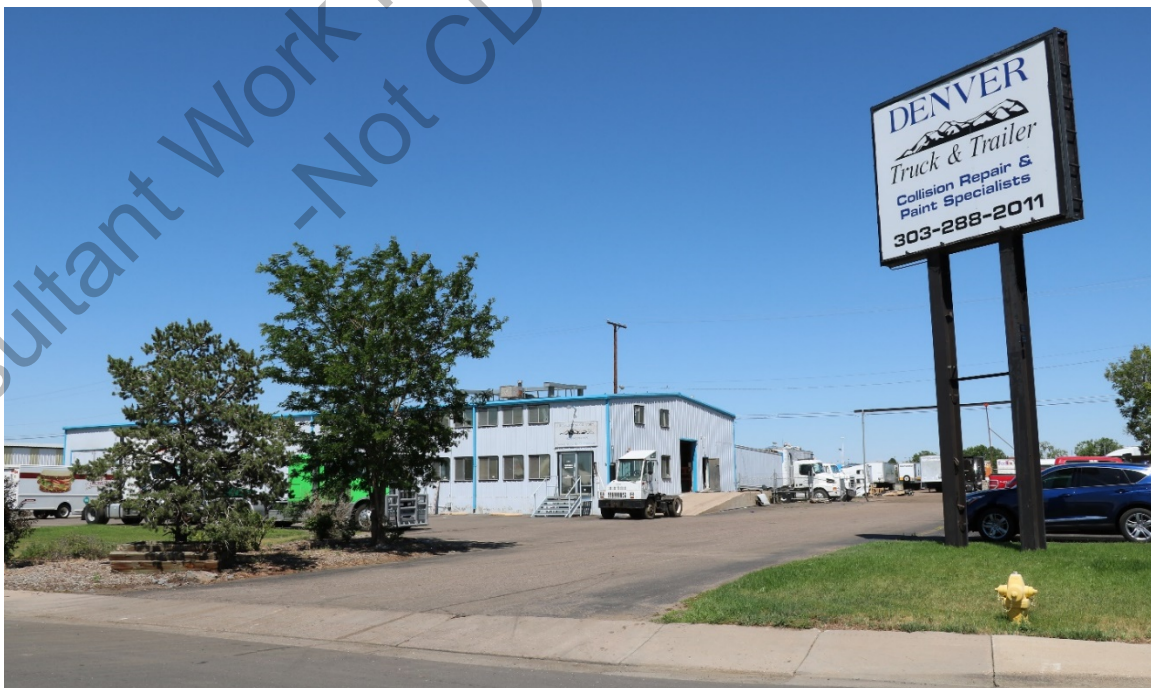
Figure 55. 5280 Newport Street facade (west) and south elevation, view facing northeast.
