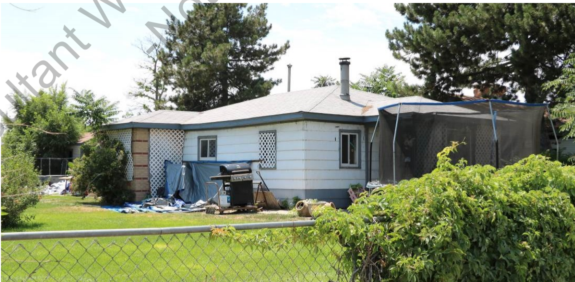
Figure 41. Marquez House, front (north) facade and side (east) elevation. View facing southwest.
