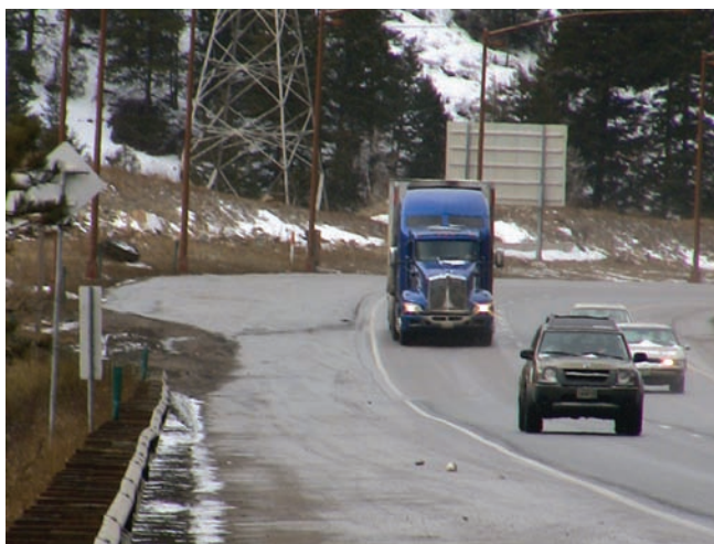
Existing chain station.
