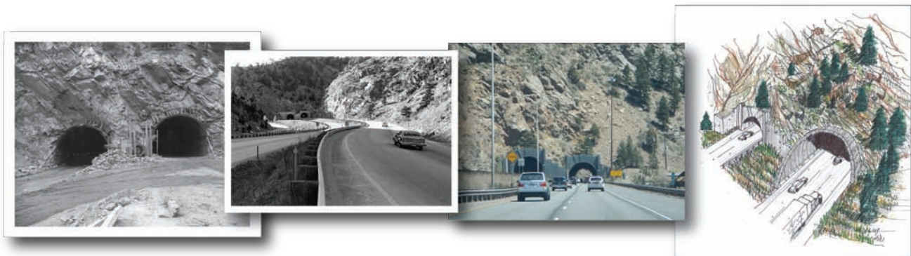
The Twin Tunnels represent the first tunneling operation on I-70. Completed in 1961, the tunnels have undergone little change since construction. The Proposed Action would widen the eastbound bore and replace its portal face with a three-dimensional façade that will help reduce the “tunnel effect” that causes drivers to slow down entering the tunnel because of their perceived (and real) narrowness. From left to right, the tunnel under construction (1959), early in its operation (1971), modern view (2012), and artist’s rendering of the Proposed Action.
