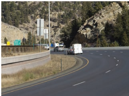
Retaining wall to improve sight distance.
