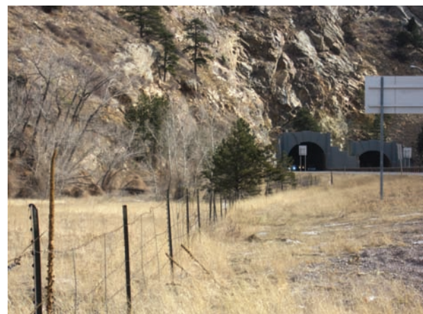
Barbed wire fencing to be replaced with wildlife-friendly fencing.
