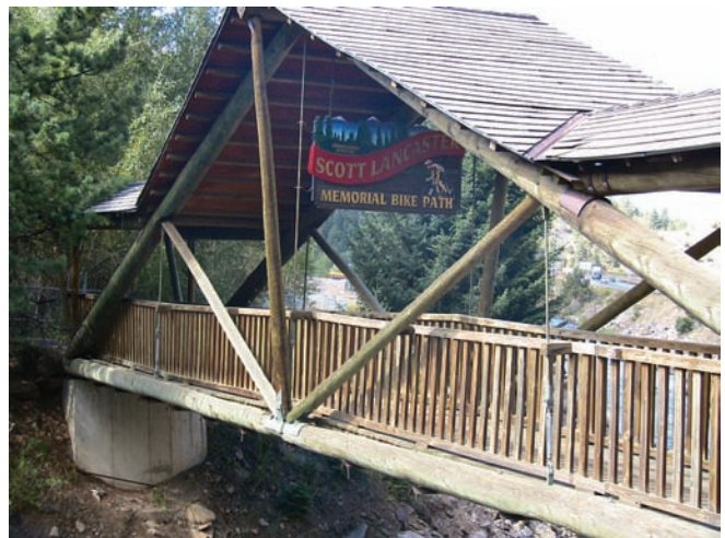
A new noise barrier installed near the Scott Lancaster Memorial Bridge will reduce noise and improve the recreational experience for users of the Scott Lancaster Memorial Trail.
