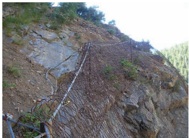
Rockfall mitigation installed under CDOT Rockfall Program.
