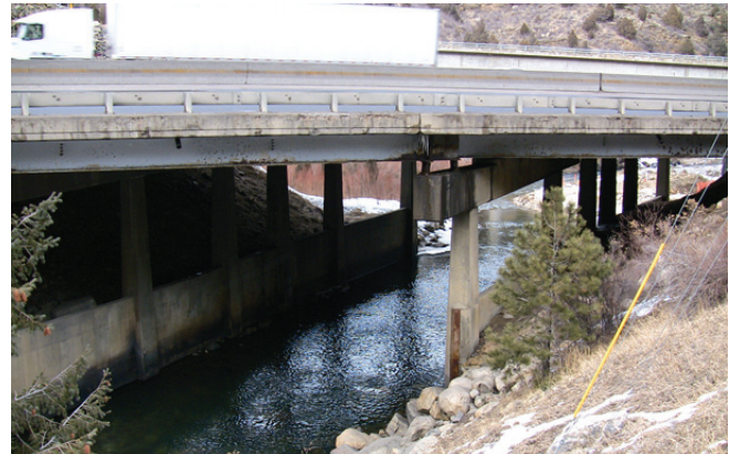
Existing bridge over Clear Creek at Hidden Valley.
