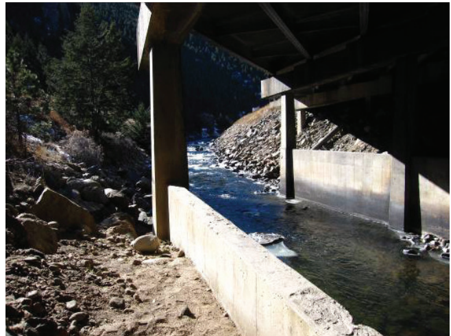
Wildlife movement/crossing area beneath Hidden Valley bridge.
