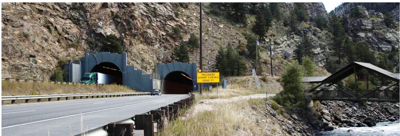
Twin Tunnels from Eastbound I-70 near Idaho Springs.
