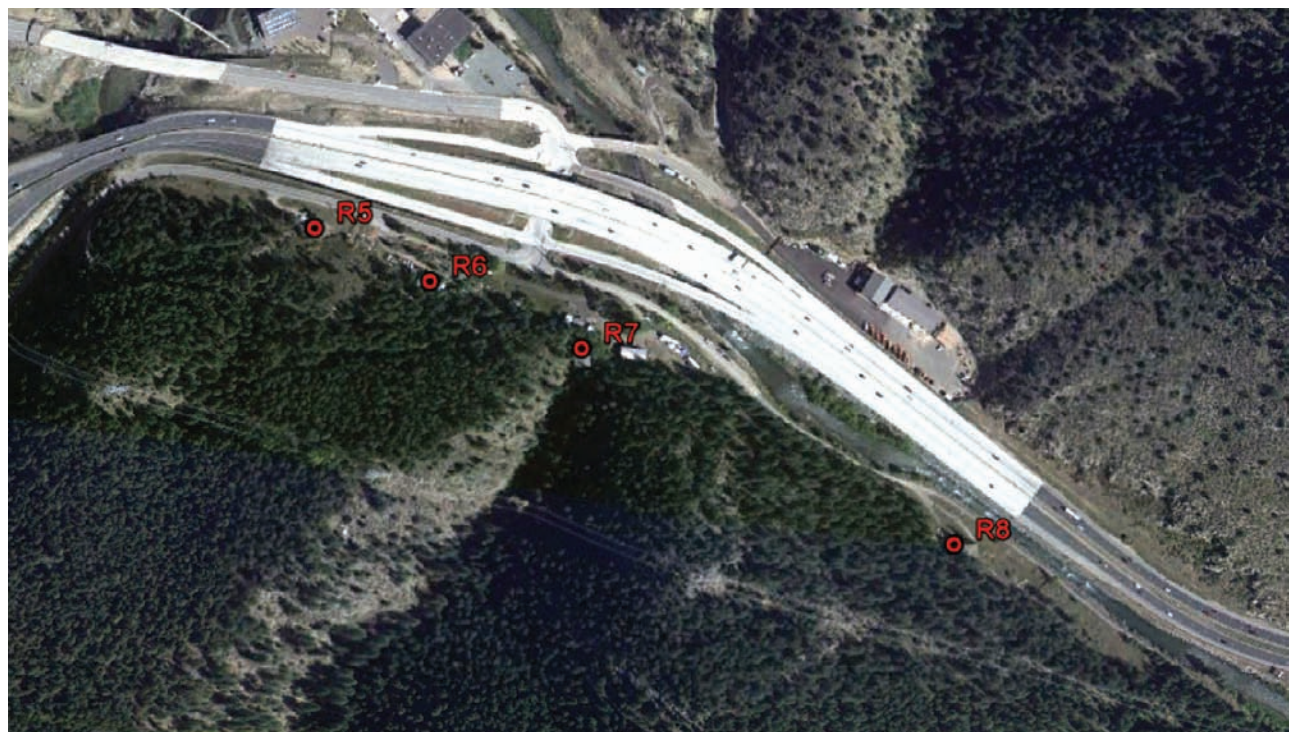
Figure 3-18. Receptor Locations East of the Twin Tunnels
