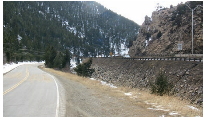
Location of proposed curve straightening. CR 314 on left, I-70 to the right.
