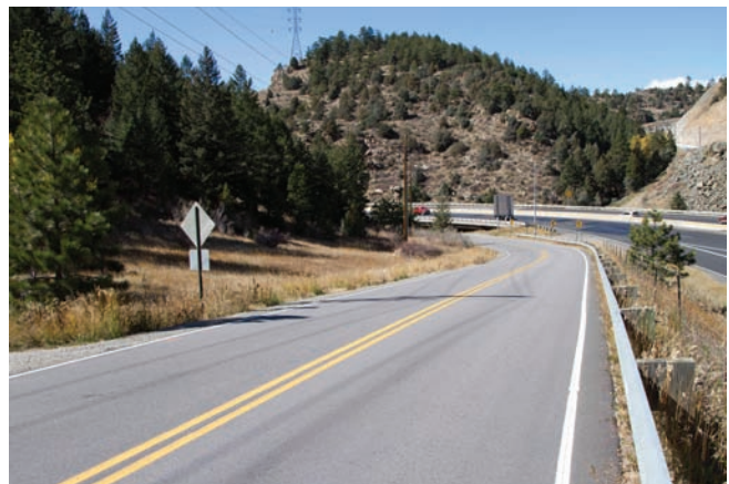
CR 314, shown to the left, is an I-70 frontage road that provides local and recreational access within the Twin Tunnels project area. CDOT is currently improving CR 314 to add a shared use path.
