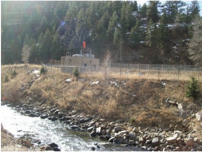
Idaho Springs Wastewater Treatment Plant storage tank area.
