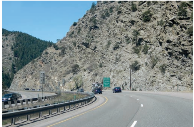
Westbound I-70 lanes are nestled against the mountainside. Flattening the westbound curves or adding lanes in the westbound direction would require significant rock cuts and/or encroachment into eastbound travel lanes and Clear Creek.
