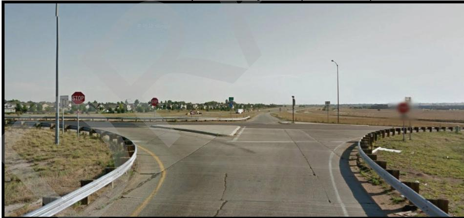
Broadside crashes were split equally between I-76 eastbound off ramp and eastbound Bromley Lane traffic failing to yield right of way at a stop sign. Similar to the westbound ramp termini, the ramp intersection is slightly skewed. With the channelized left turn from the ramp, the stop sign placement to be further back for the eastbound I-76 off ramp and eastbound Bromley approaches.
