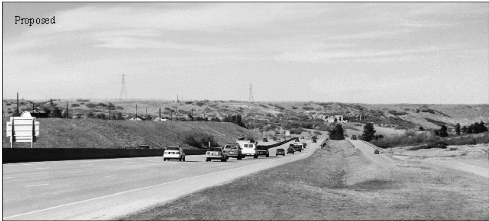
Figure 5.10 illustrates the existing and proposed view (Preferred Alternative and Other Alternative) of I-25 at Castle Pines Parkway, looking north. The proposed view shows the existing noise wall (recommended in the Climbing Lanes, Phase I project) and I-25 widened to four lanes in each direction
