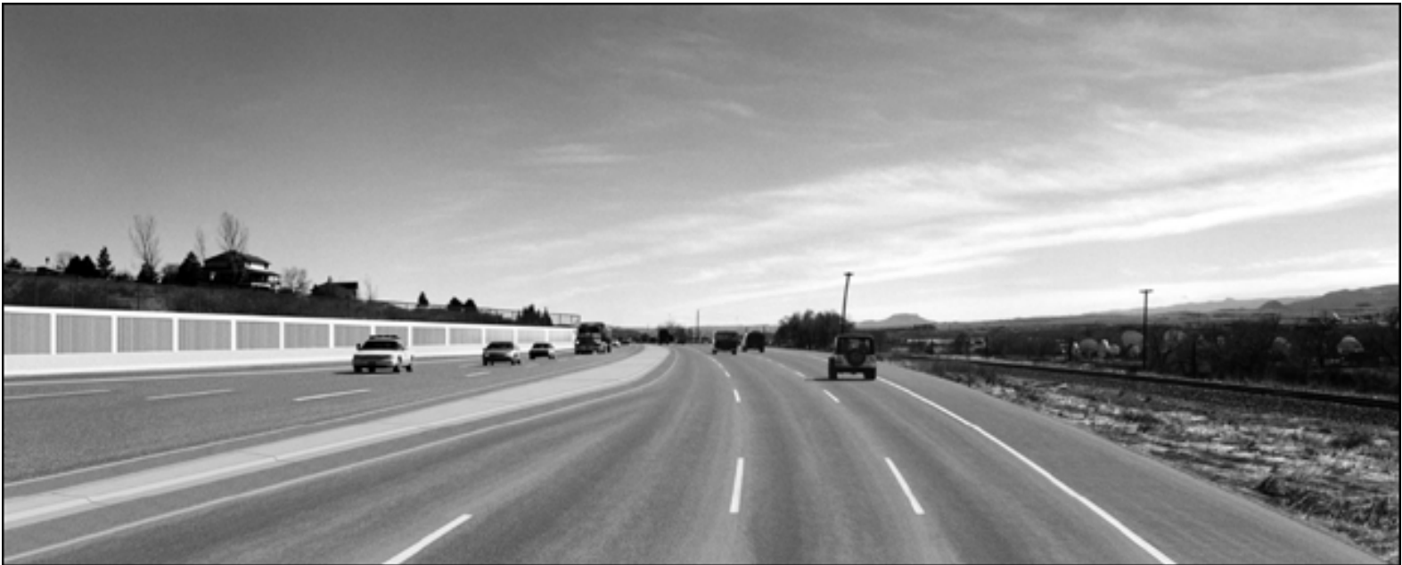
Figure 5.16 Existing and Proposed View of US 85 Corridor at SH 67 (looking north) (Preferred Alternative and Other Alternative)
