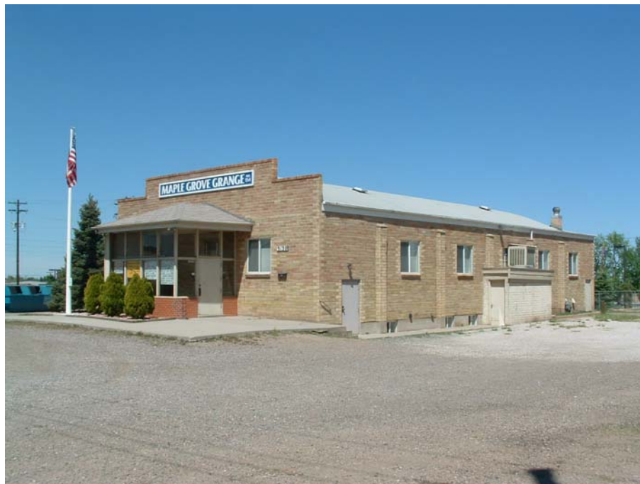
Figure 4-20 Maple Grove Grange Building (5JF4327)
