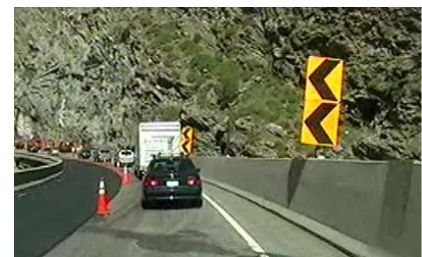
The nature of Floyd Hill's steep, two-mile long, 6% westbound downgrade has resulted in serious traffic crashes in the past. A Reversible Lane could result in a 2.5-mile westbound backup, or to the top of Floyd Hill, if implemented.
