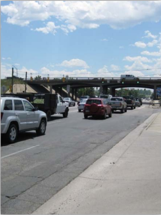
Kipling Street at eastbound I-70 ramps intersection
