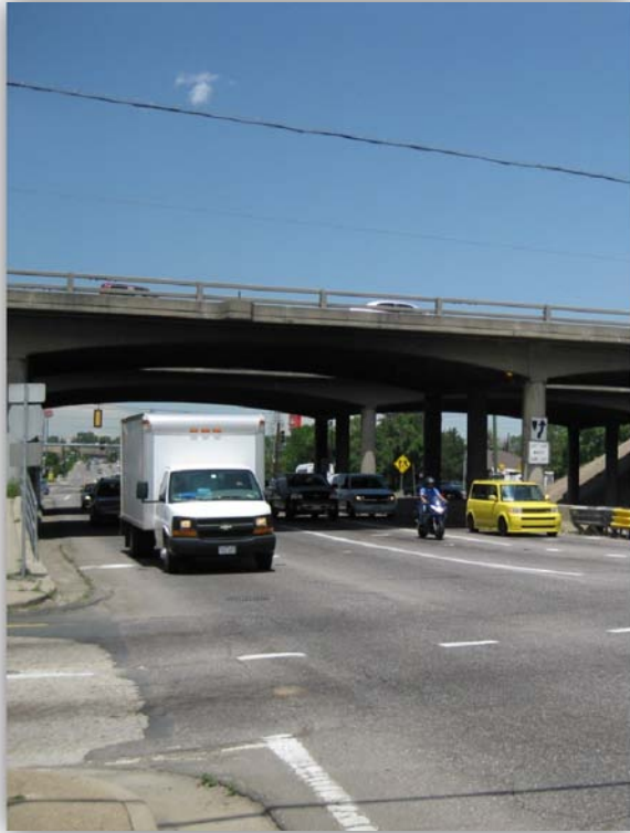
Looking north along Kipling Street towards I-70
