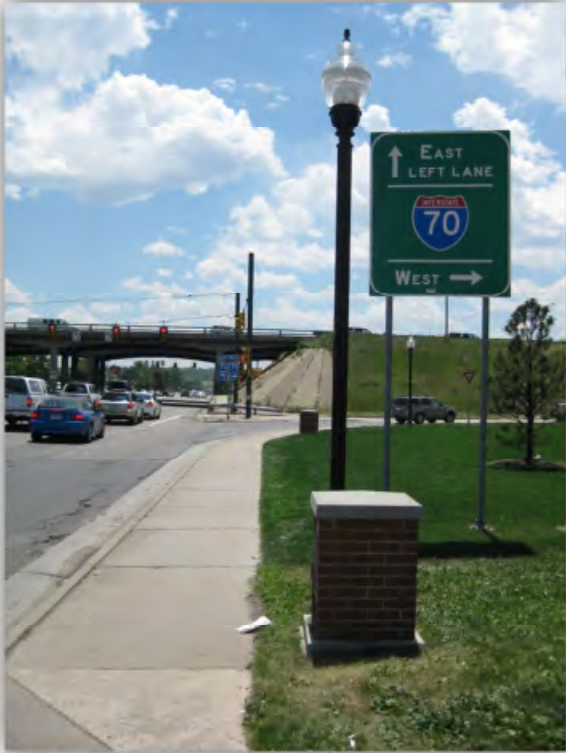
Looking south along Kipling Street towards I-70
