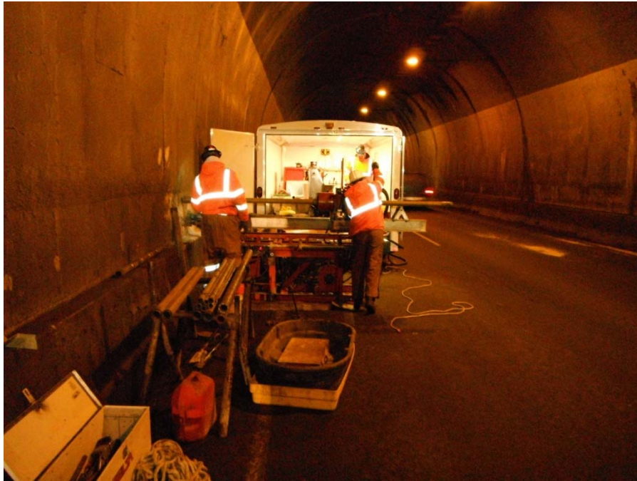
Site setup and location for YA-T-01 in left/north lane of eastbound I-70. Total depth 20.1 ft, horizontal. This photo is also representative of borings YA-T-04 (19.3 ft, horizontal) and YA-T-05 (20.0 ft, horizontal)
