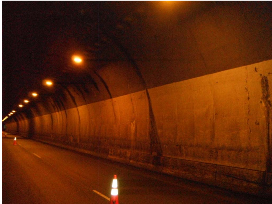
Looking east at right/south lane of eastbound tunnel, midsection.
