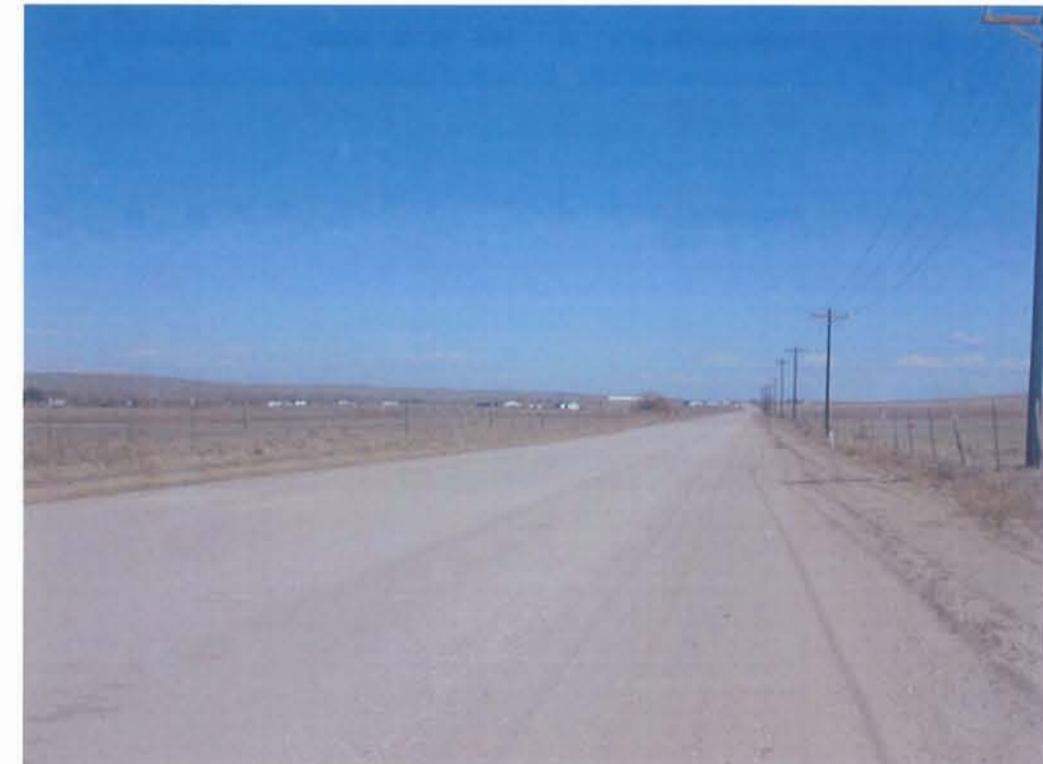
Figure 13-3--Kiowa-Bennett Road in Elbert County
