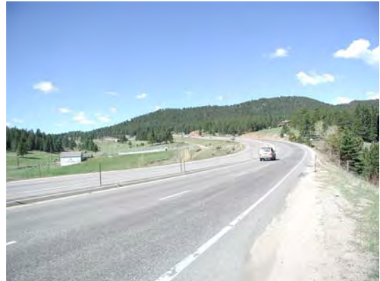
Shaffers Crossing, southbound US 285, MP 231
