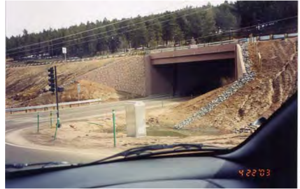
Grade-separated intersection with underpass at Conifer. Note vertical face abutments of the bridges placed near the edge of shoulder
