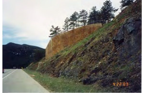
Retaining wall adjacent to US 285 east of Aspen Park
