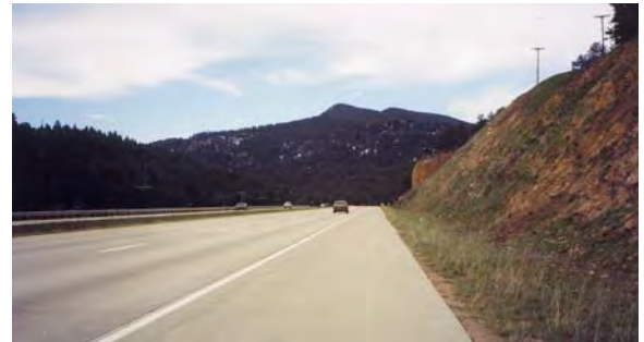
Cut slope adjacent to US 285 east of Aspen Park
