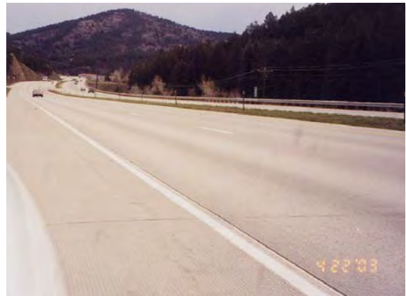
Completed US 285 phase east of Aspen Park
