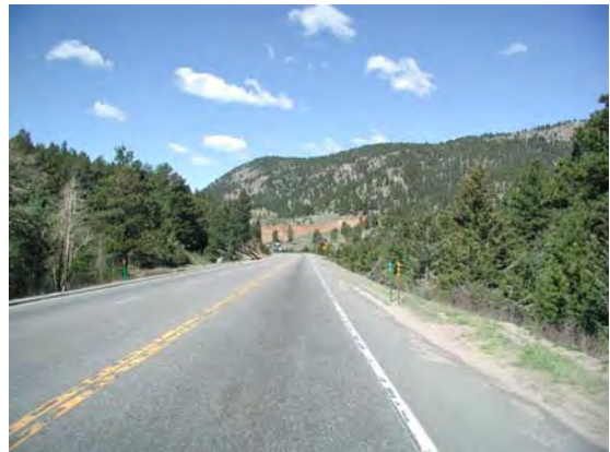
US 285 southbound, between Pine Junction and Deer Creek
