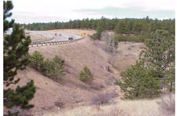
Roland Gulch fill slope and culvert, view to west.
