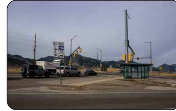
Curb cuts at US 6 and Jefferson County Parkway
