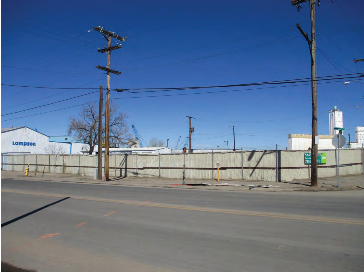
5AM4076_3.jpg: Looking northwest at 5AM.4076 from E. 60 th Ave. (March 3, 2021)
