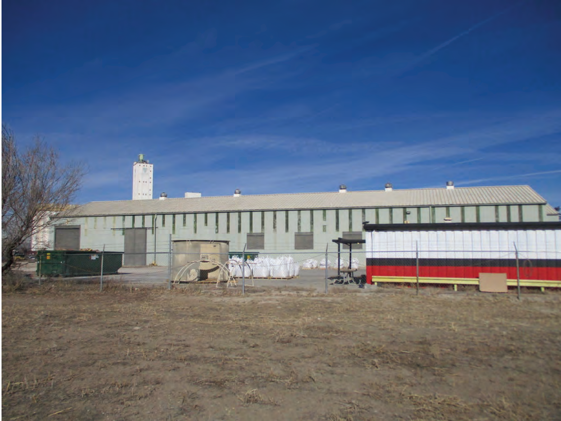
5AM4077_4.jpg: Looking north at 5AM.4077 main building and Building B from parking lot on adjacent site (January 24, 2020)
