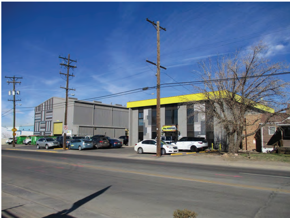
5AM4075_2.jpg: Looking northwest at 5AM.4075 from E. 60 th Ave. (January 24, 2020)
