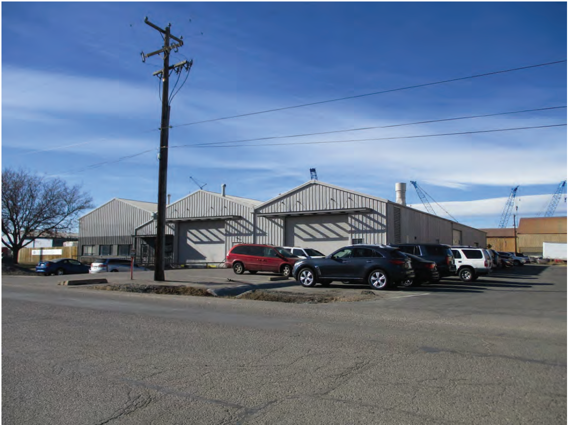
5AM4080_1.jpg: Looking west at 5AM.4080 from Clermont St. (January 24, 2020)
