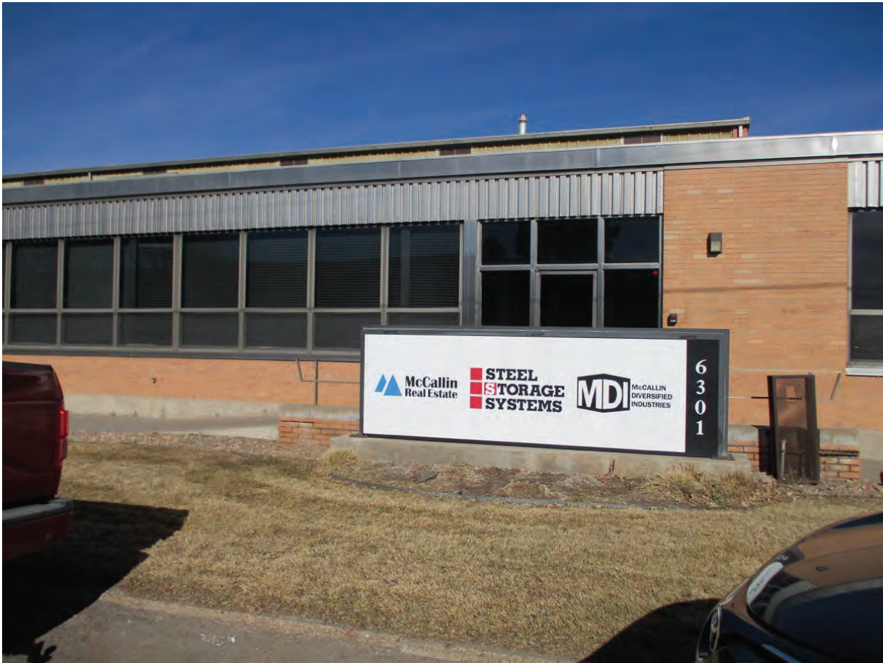
5AM4083_3.jpg: Looking north at 5AM.4083 from E. 63 rd Ave. (January 24, 2020)
