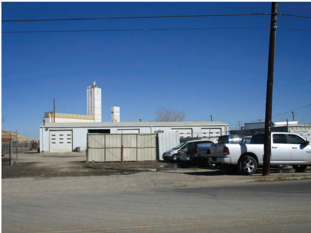
5AM4076_2.jpg: Looking north at 5AM.4076 from E. 60 th Ave. (March 3, 2021)
