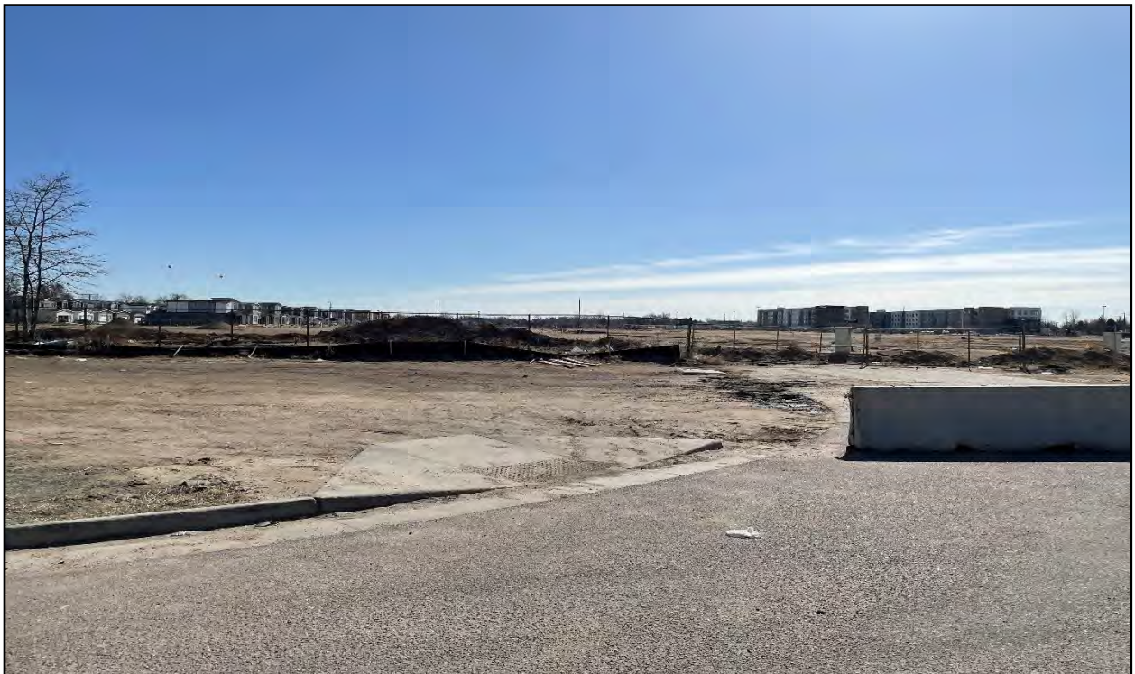
Photo 22: View of the Mile High Greyhound Park development from Highway 2 facing east.
