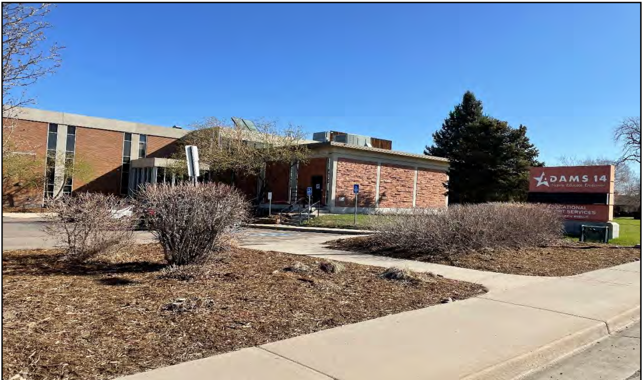
Photo 12: View of the Adams County School District Educational Support Services building on E 60 th Ave facing northeast.
